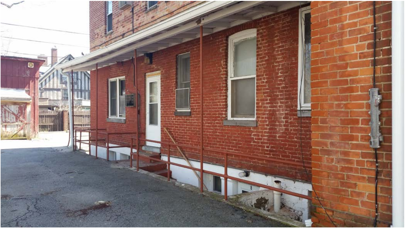
Figure 2: North side, east entrance
