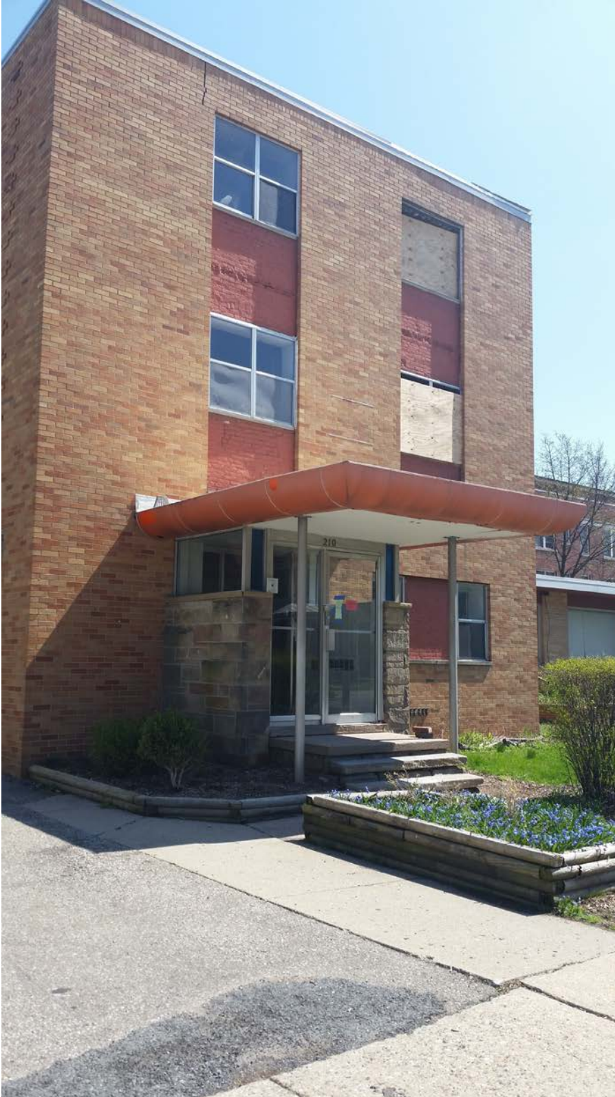
Figure 5: West side, north entrance
