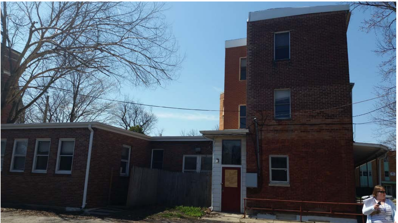
Figure 3: East side, north entrance
