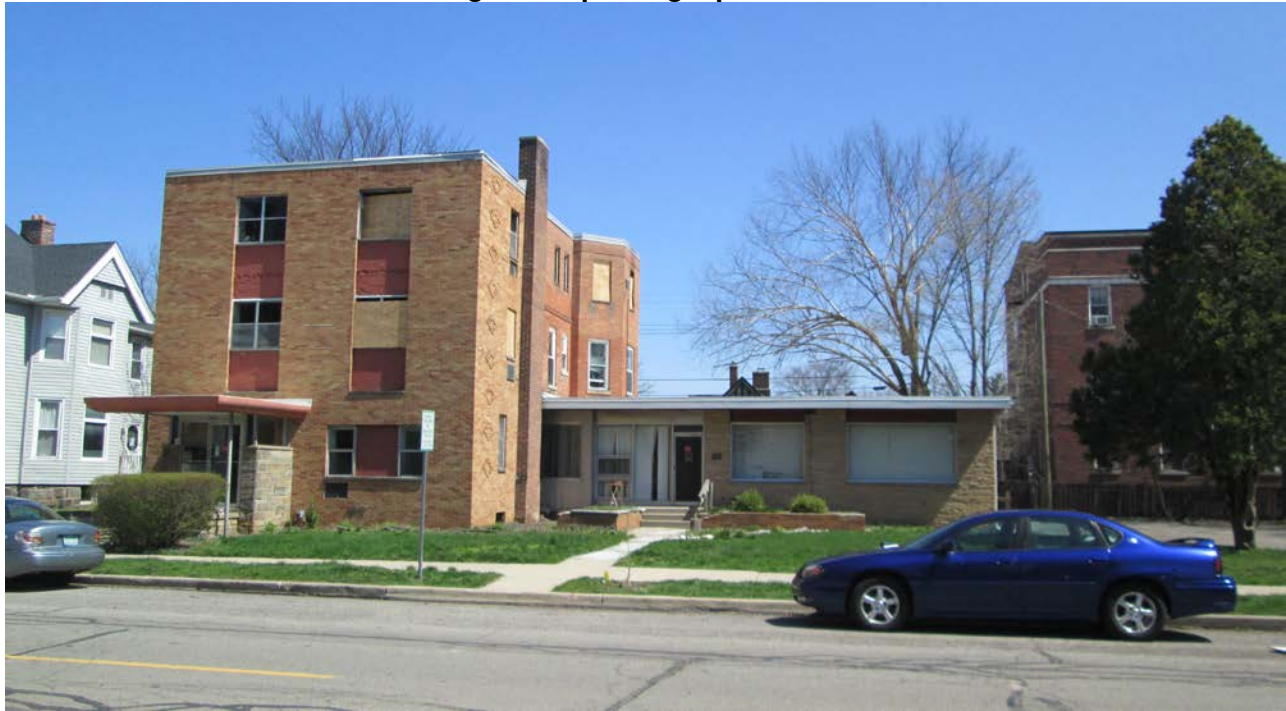
Figure 3: photograph of site
