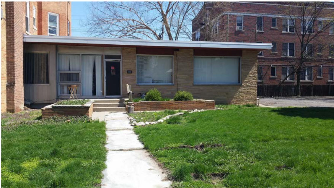
West side, south entrance
