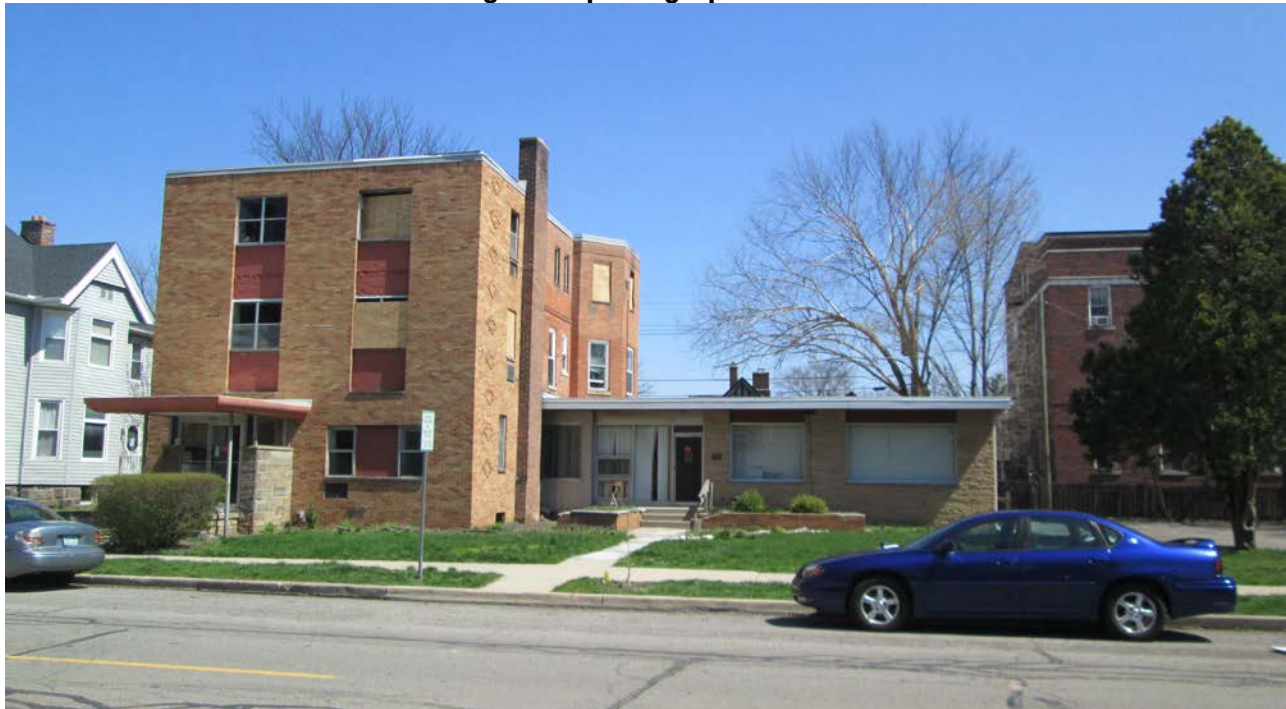
Figure 3: photograph of site
