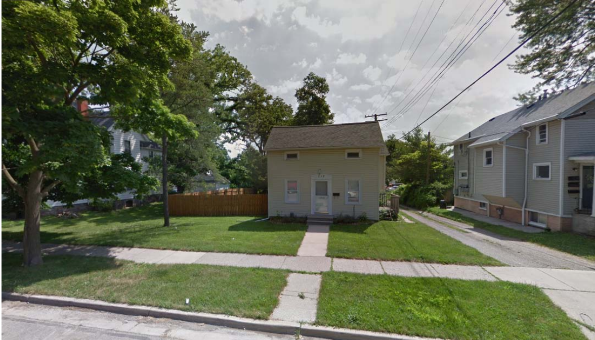
Figure 3: photograph of site Google Street View (July 2018)
