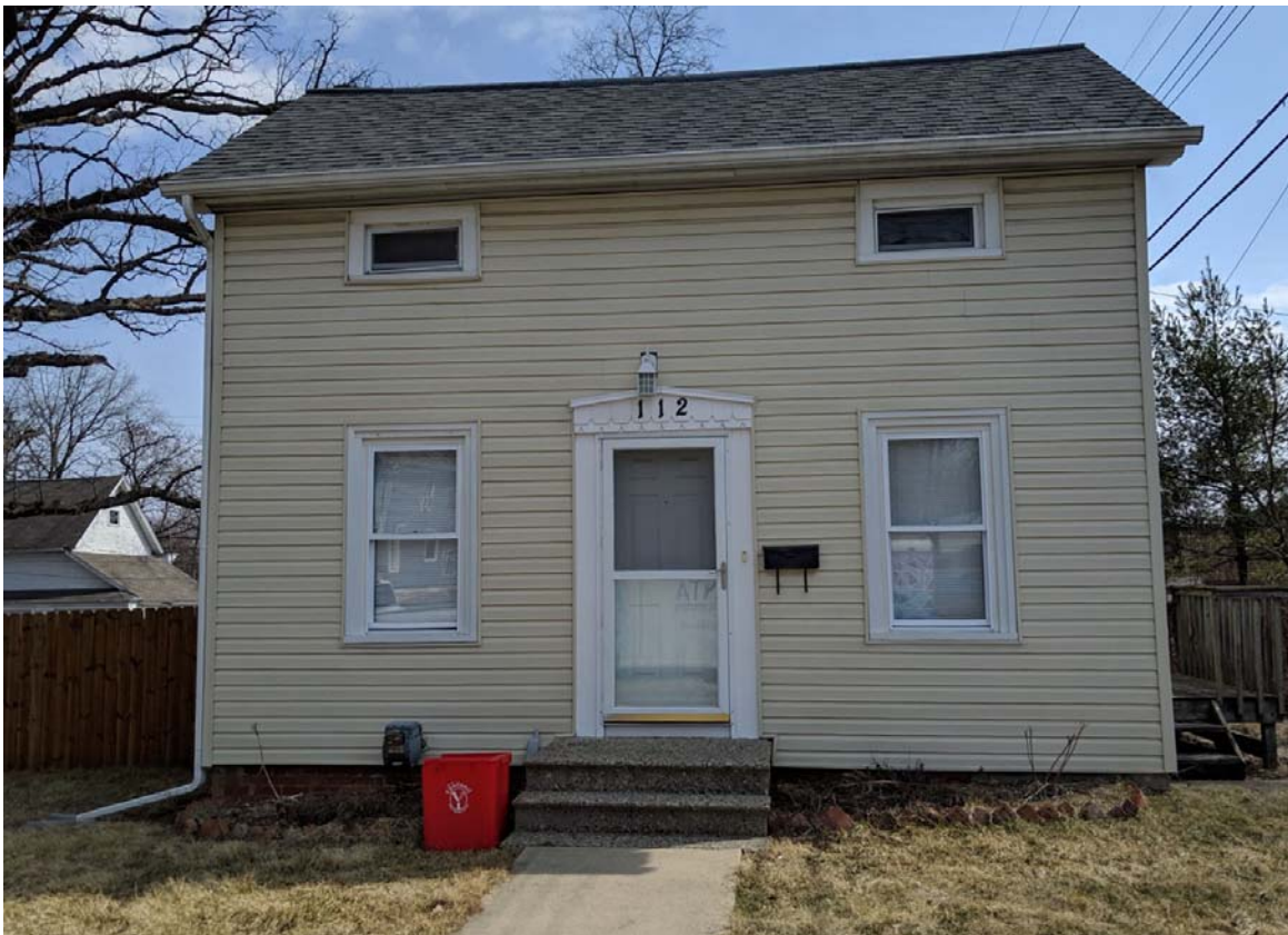
Figure 4-8: photographs of site (March 2019)
