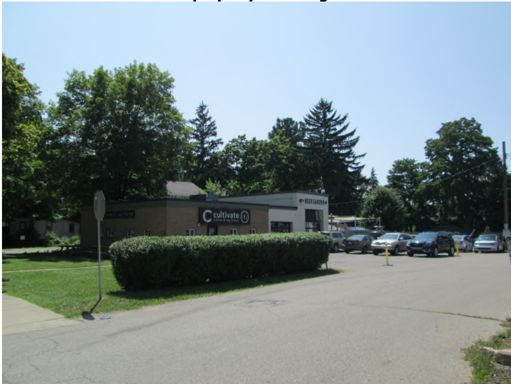
Facing southwest to north and west elevations.
