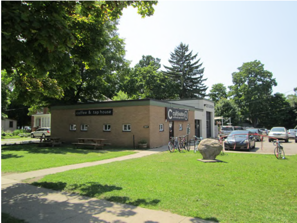
Facing southwest to north and east elevations.
