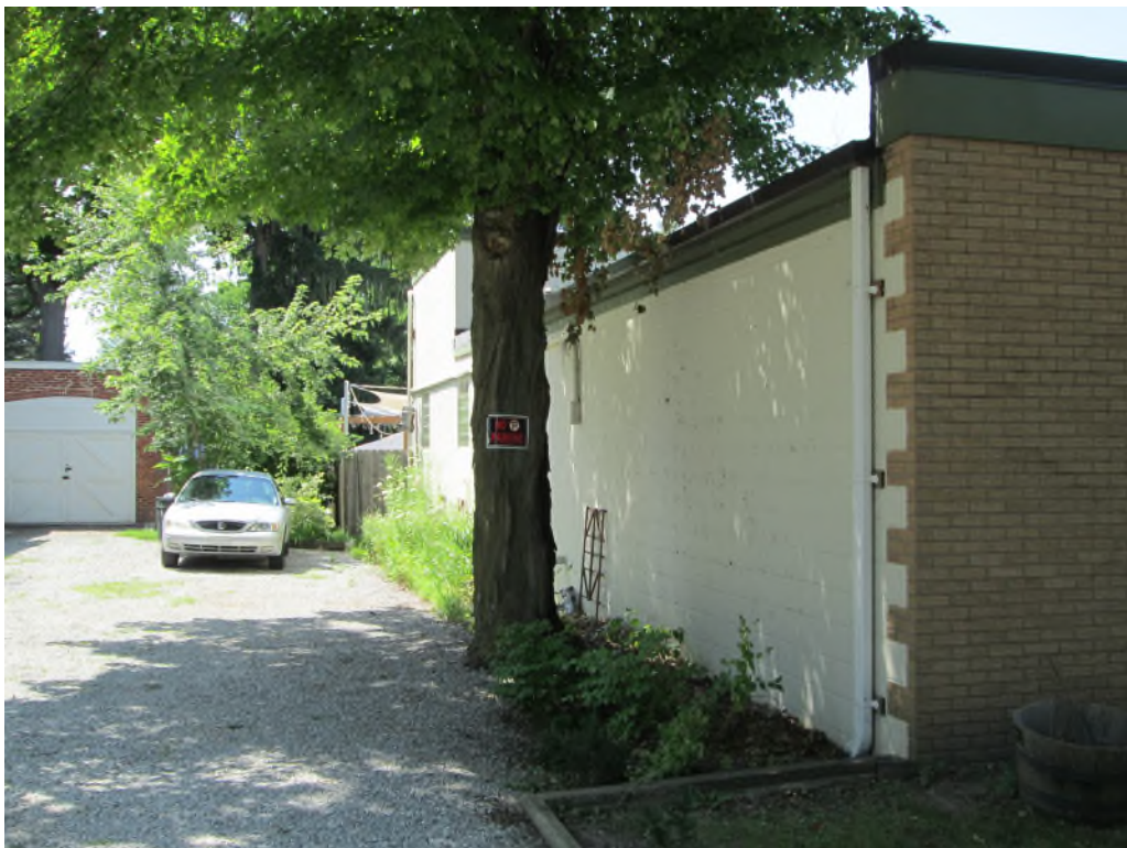
Facing west-northwest along south property boundary.
