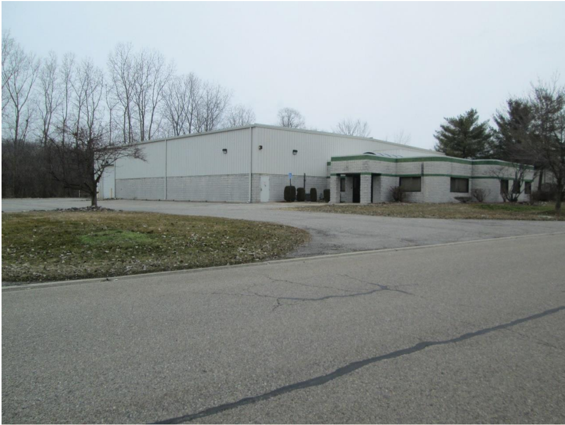
Figures 6-8: Photographs of Building and Site (March 11, 2020)
