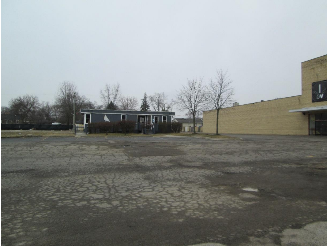
Figures 9-10: Modular Office Building and Parking Lot (March 11, 2020)
