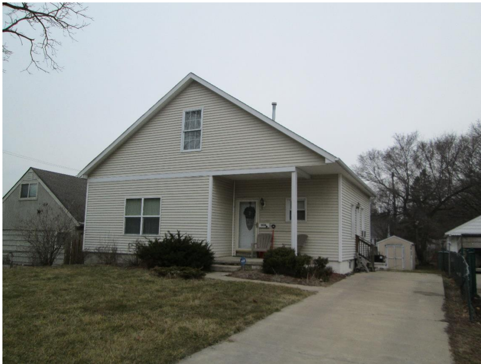
Figure 2: 1226 S Congress, facing northwest (March 2020)
