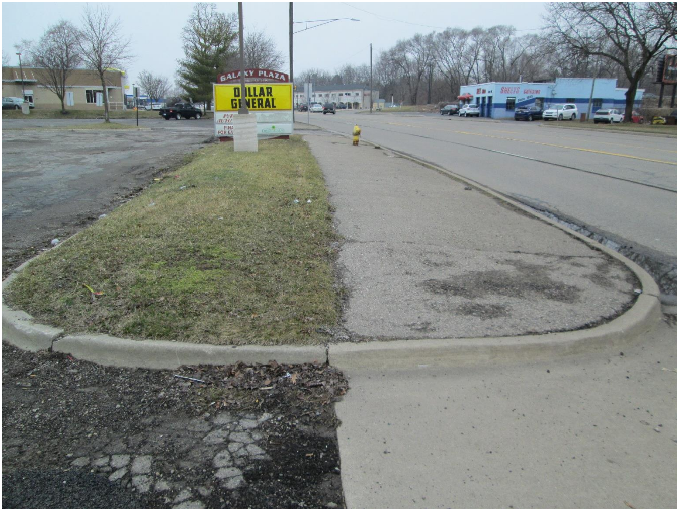
Figures 6-8: Photographs of Sidewalk (March 11, 2020)
