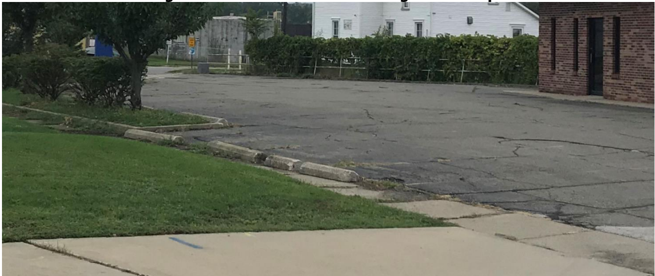
Figure 8: Zoomed Photo of Existing Wheel Stops
