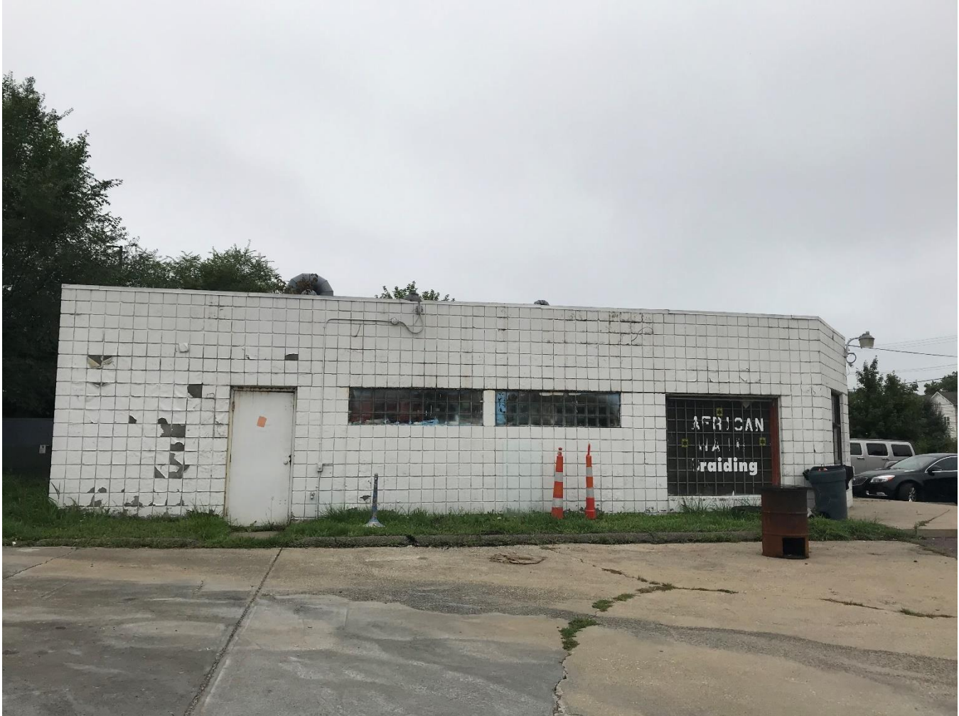
Figure 8: Photo of Building (Side Elevation, September 2020)
