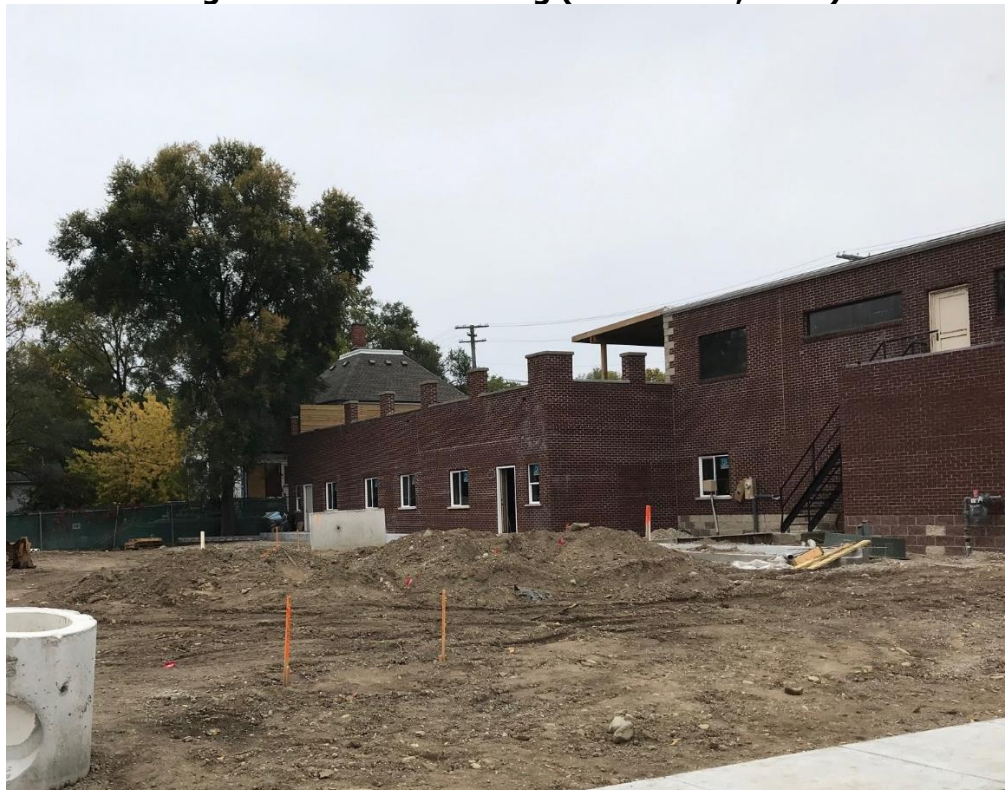
Figure 5: Rear of building (October 14, 2020)
