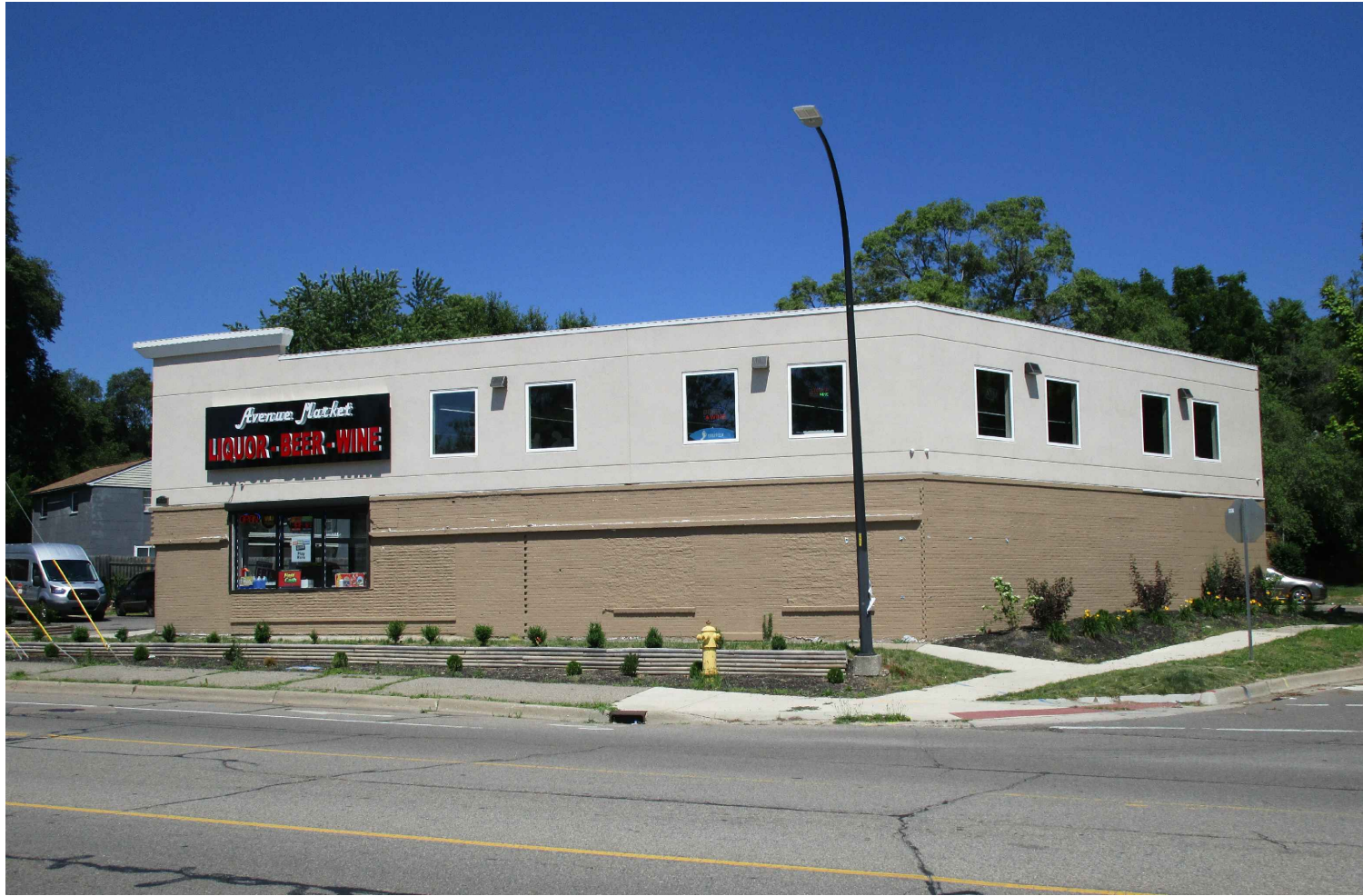
1 E100 Existing Image - Front Facade
