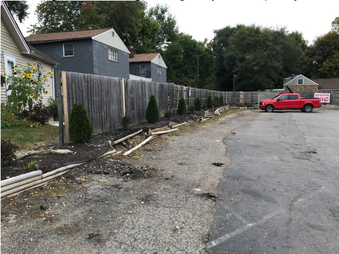
Figure 14: Crumbling retaining wall (October 14, 2020)
