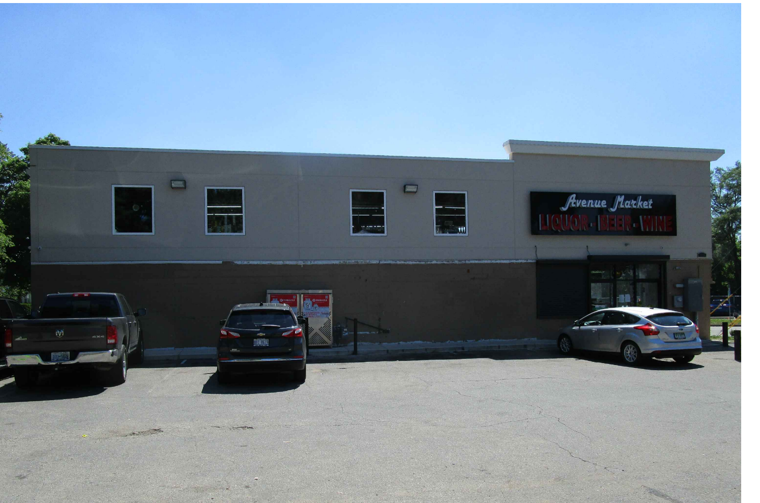
4 E100 Existing Image - Parking Lot Facade
