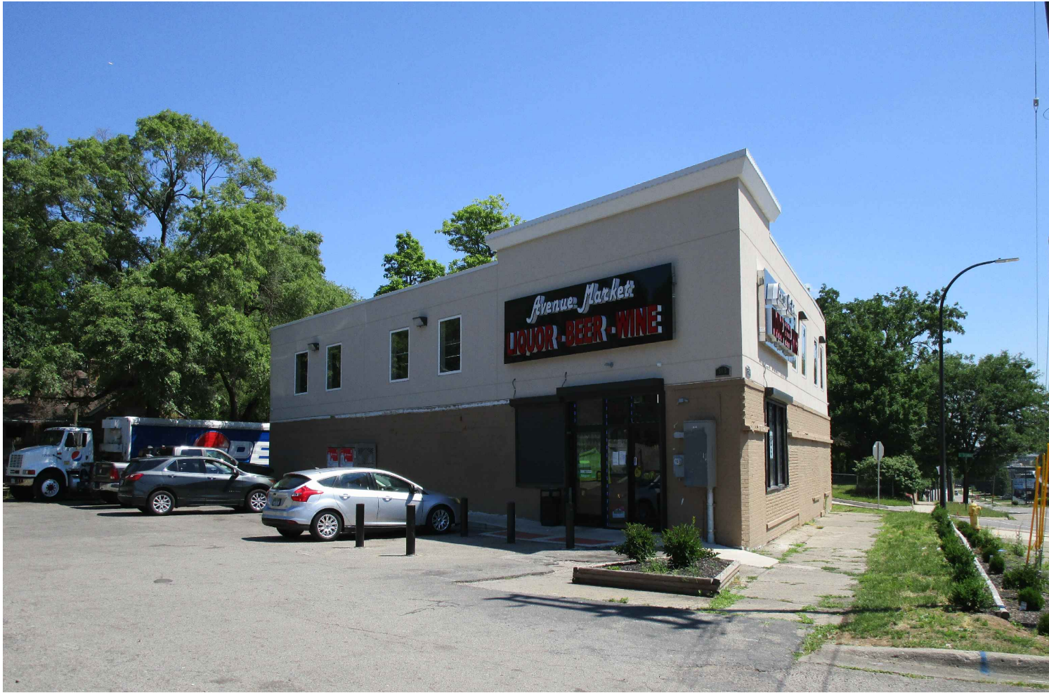
2 E100 Existing Image - Entry Facade
