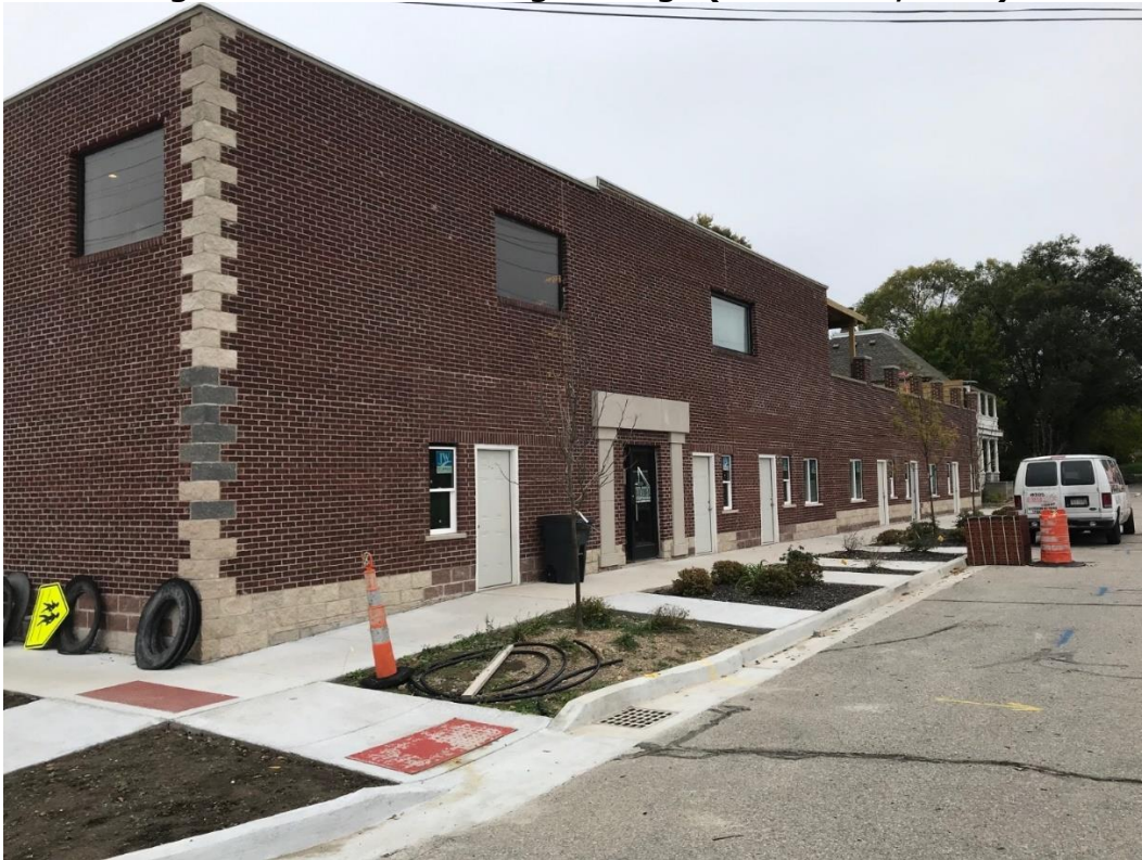
Figure 4: N. Park building frontage (October 14, 2020)
