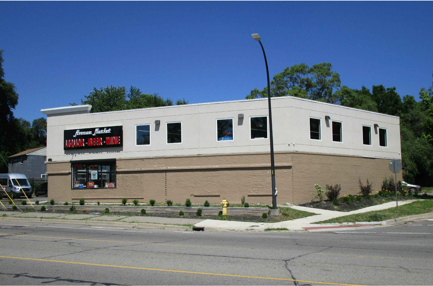
1 E100 Existing Image - Front Facade
