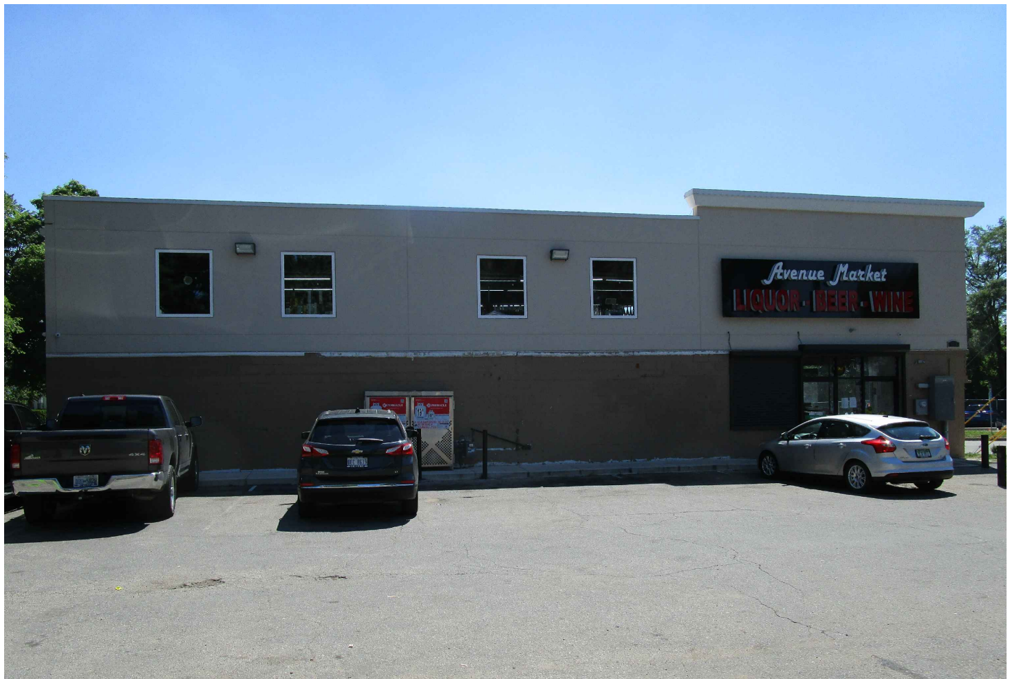
4 E100 Existing Image - Parking Lot Facade
