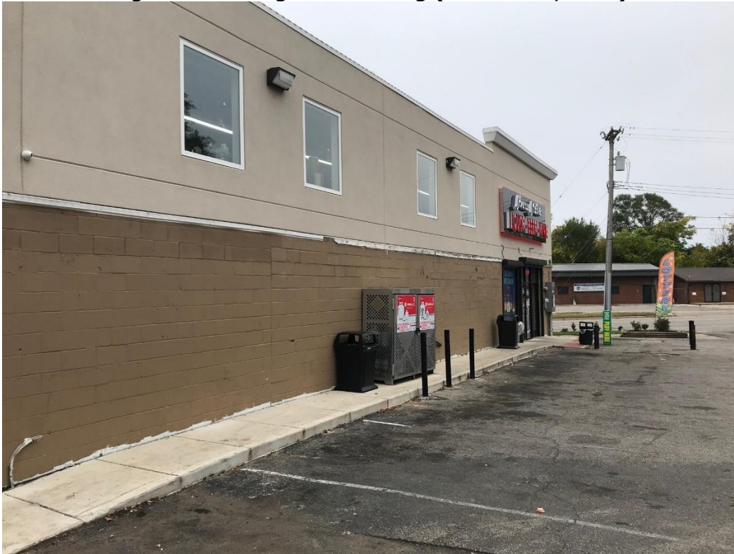
Figure 7: Parking near building (October 14, 2020)
