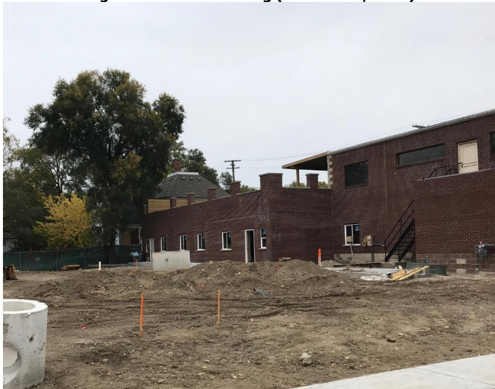
Figure 5: Rear of building (October 14, 2020)
