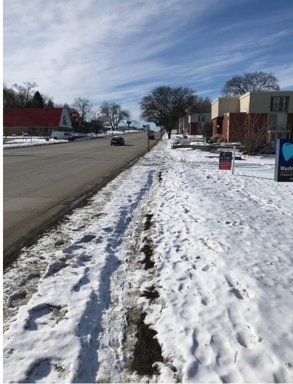
Figure 8: Lack of Front Sidewalk
