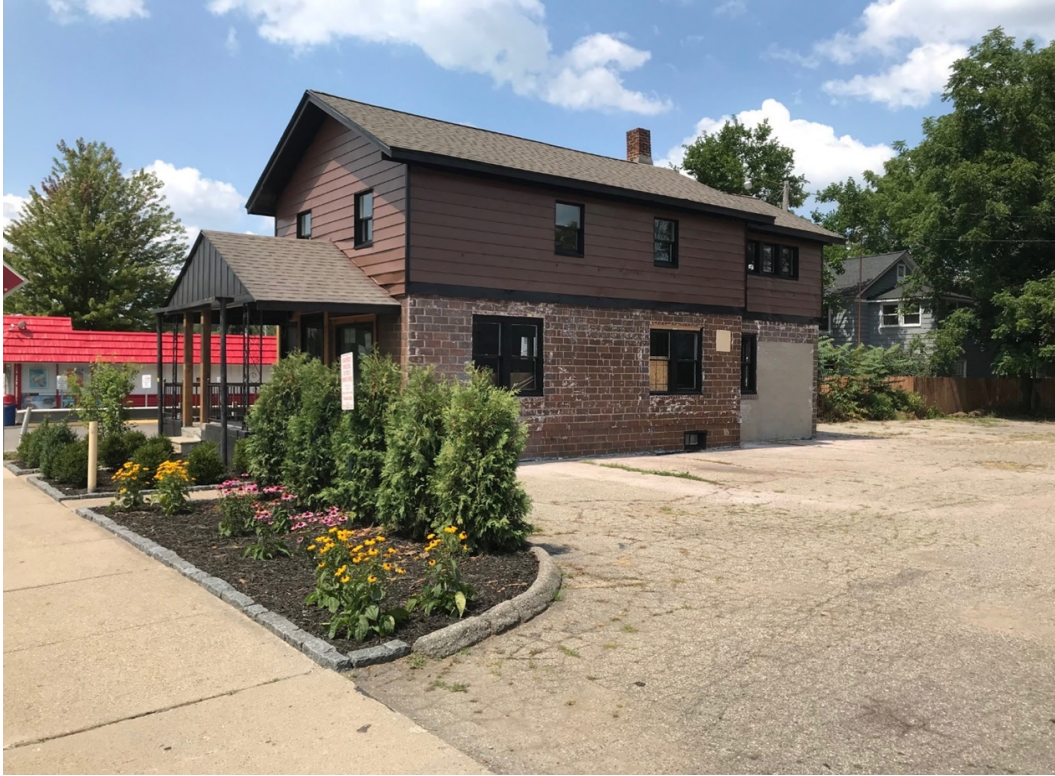
Figure 4: East Side of Site (August 4, 2021)
