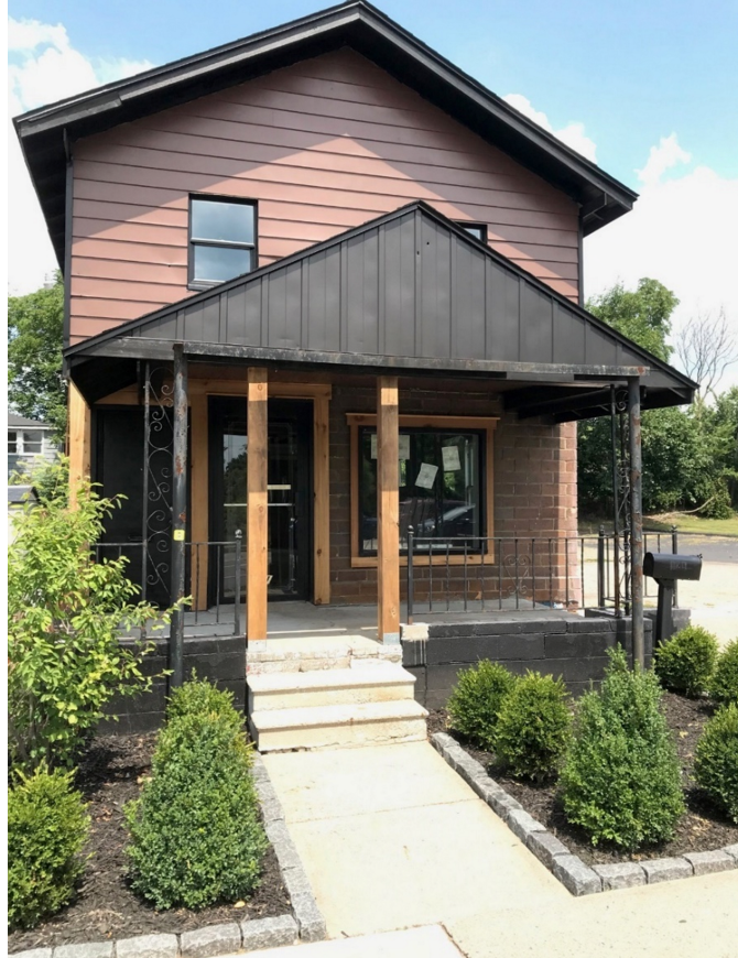
Figure 7: Front Building Façade (August 4, 2021)
