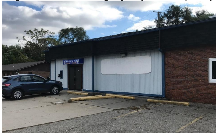
Figure 5: Front of Building Façade (October 12, 2021)
