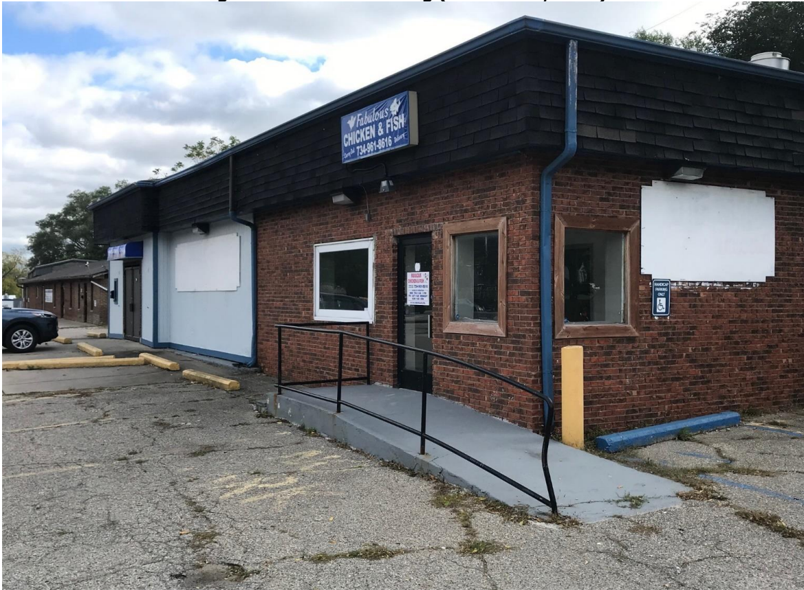
Figure 2: Front of Building (October 12, 2021)
