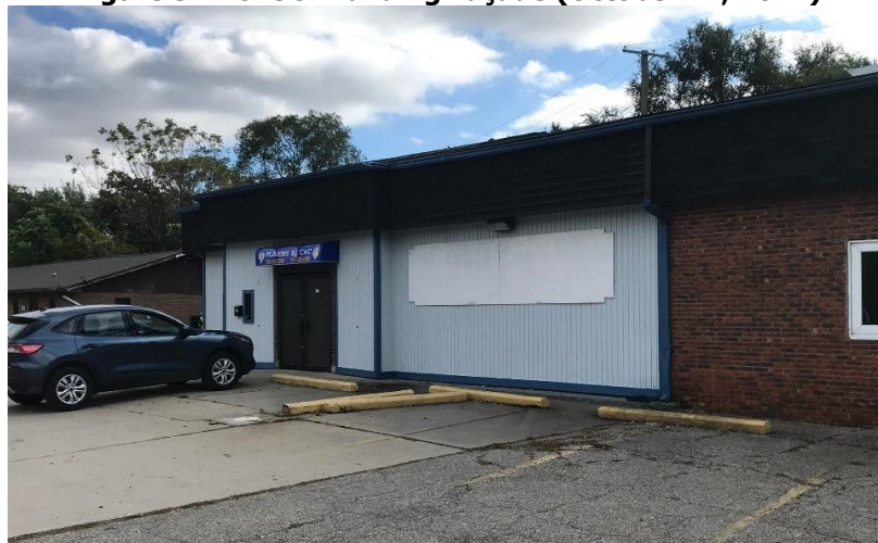
Figure 5: Front of Building Façade (October 12, 2021)
