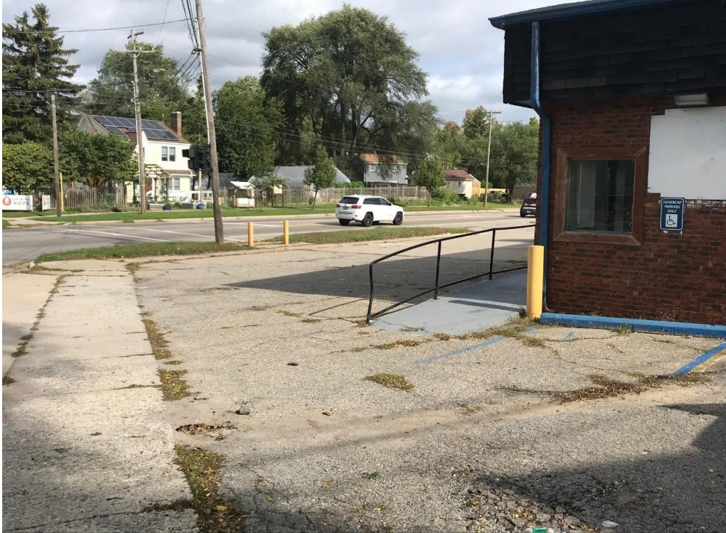
Figure 9: Side-Street Sidewalk and First Ave Curb-cut (October 12, 2021)
