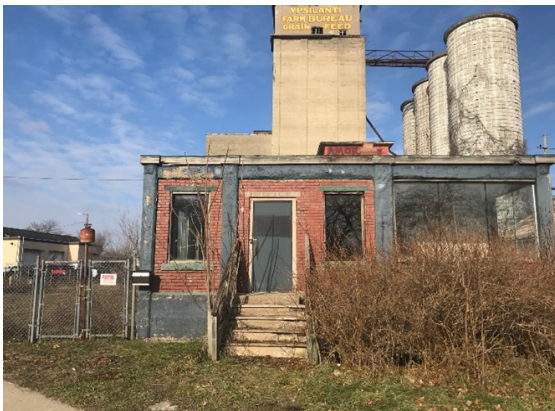
Figure 5: Existing Building "A" (December 8, 2021)
