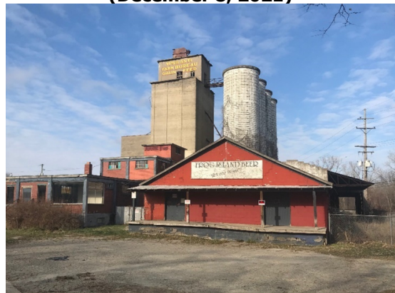
Figure 6: Existing East Building to be Demolished (December 8, 2021)
