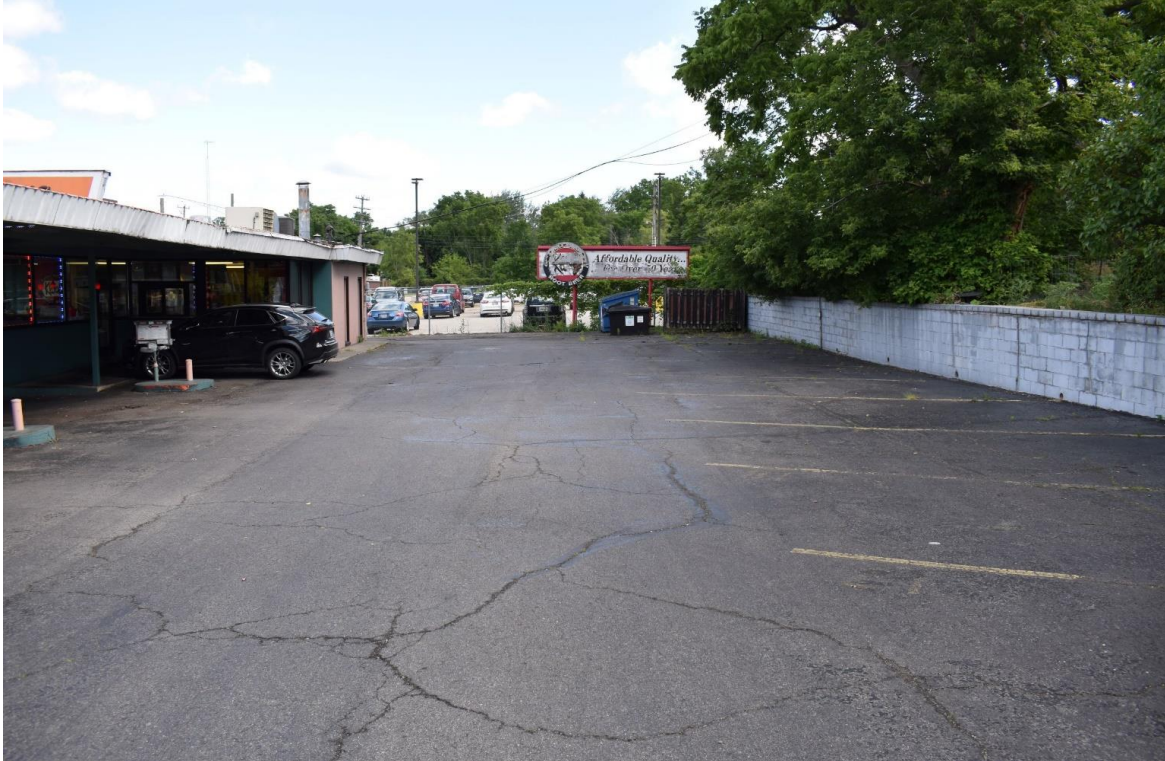
Figure 10: East Side of Parking Lot and Retaining Wall (July 12, 2022)
