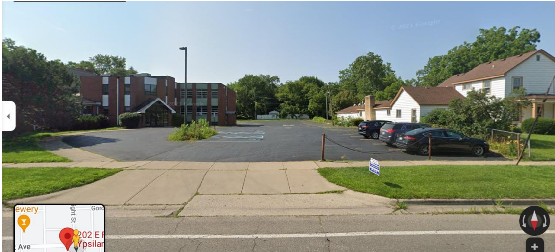
Figure 4: Church and parking lot at 218 E Forest facing south. (Google, July 2021)
