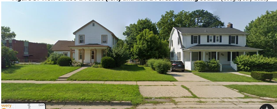
Figure 3: View of 206 E Forest (left) and 202 E Forest looking south. (Google, July 2021)
