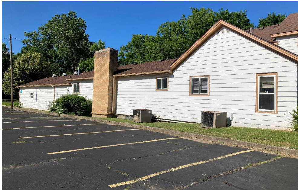
Figure 5: East side of 206 E Forest from the church parking lot, looking southwest. (June 2022)
