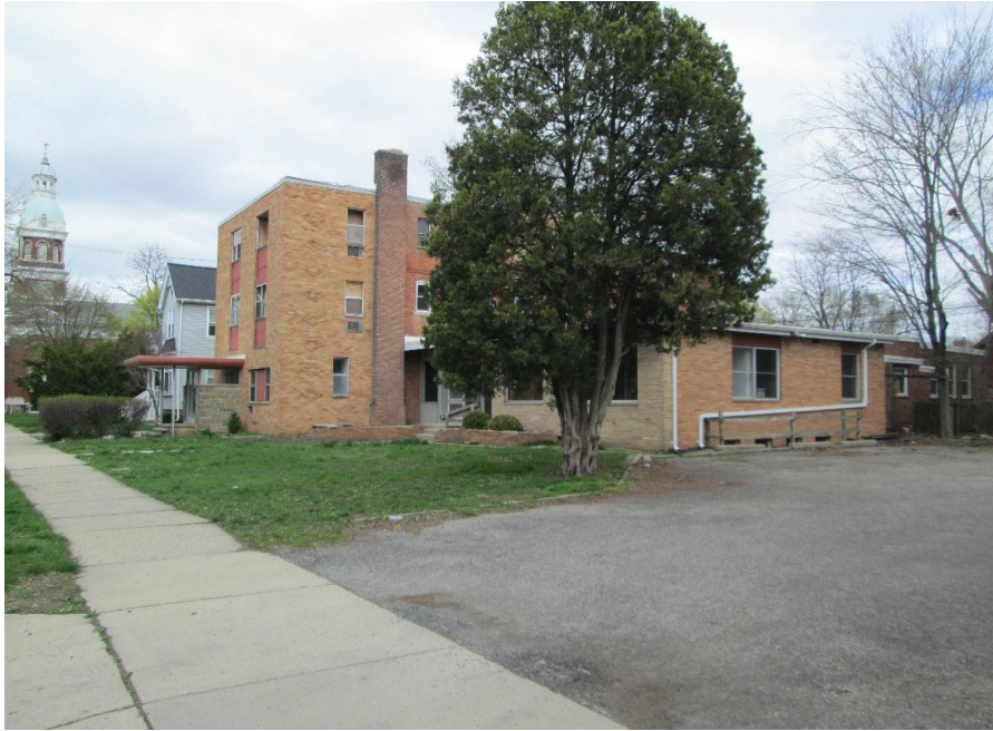
206-210 N. Washington, 2019. Photo looking northeast to façade and south elevation.
