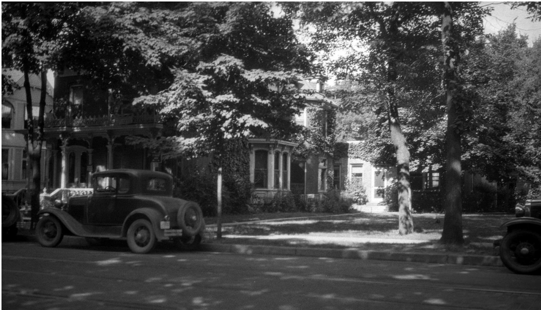
206-210 N. Washington, ca. 1930. Photo looking northeast to facade and south elevations. Note the one-story office addition.
