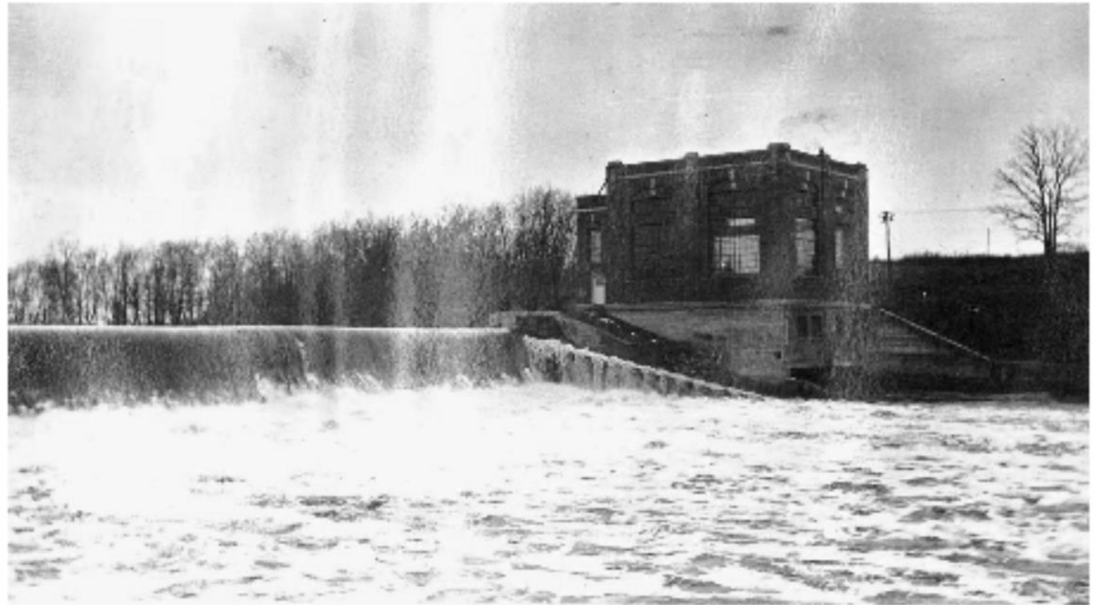
Photograph 3: View of Dam spillway
