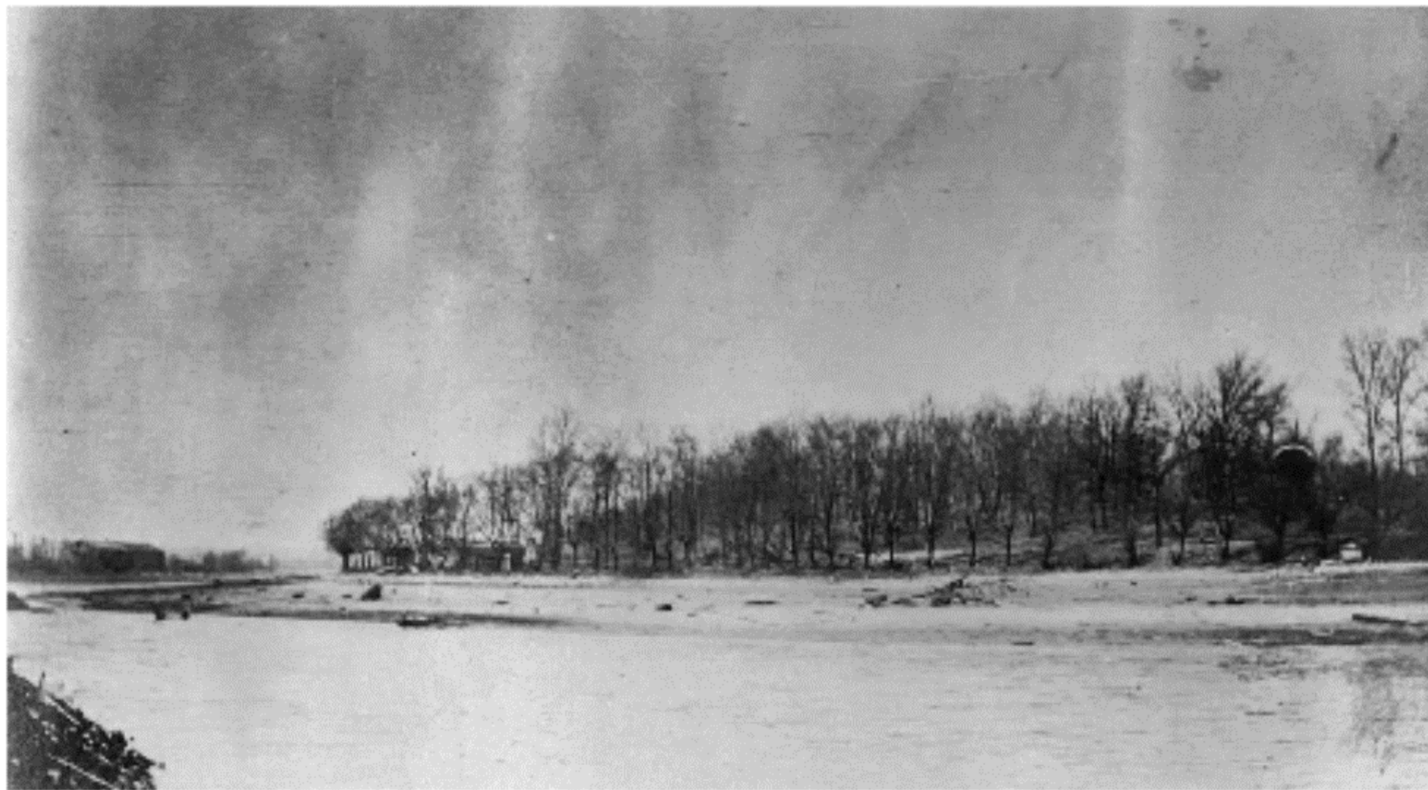
Photograph 1: View of Dam site
