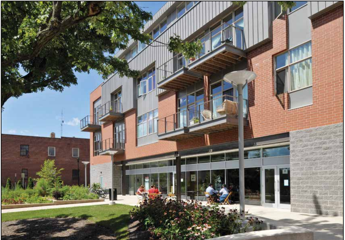
Oberlin's East College Street Project is expected to receive LEED Neighborhood Certification. Photo by Kevin Reeves for Oberlin College.
