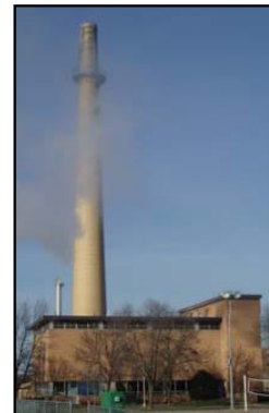
UW-Eau Claire's Coal-fired Power Plant
