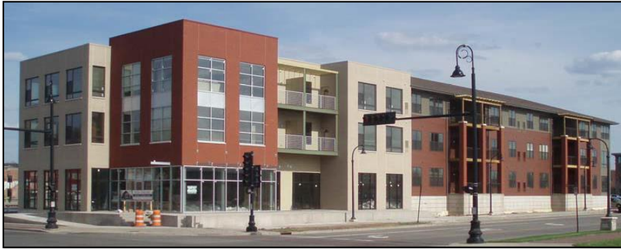
Mixed use building along Phoenix Park
