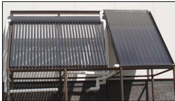
Solar hot water heating at Badger State Inc.
