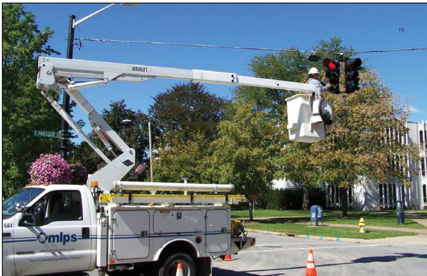
OMLPS replacing traffic lights with LED leading to a two-thirds reduction in energy use.
