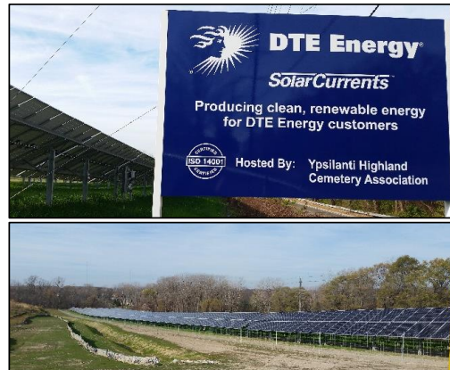
Figure 3. DTE Energy solar array located on land owned by Highland Cemetery. Source: City of Ypsilanti.
