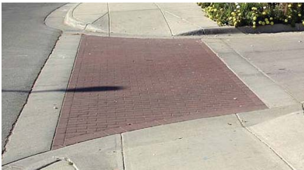
Figure 27: Driveway Apron Example
