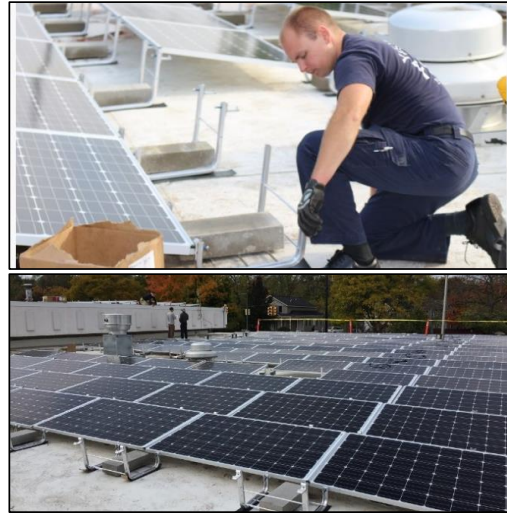
Figure 2. Solar array Installation on City of Ypsilanti Fire Station. Source: solarypsi.org
