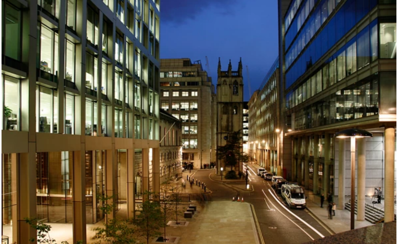
The London Wall road. Photo by David Bank.
