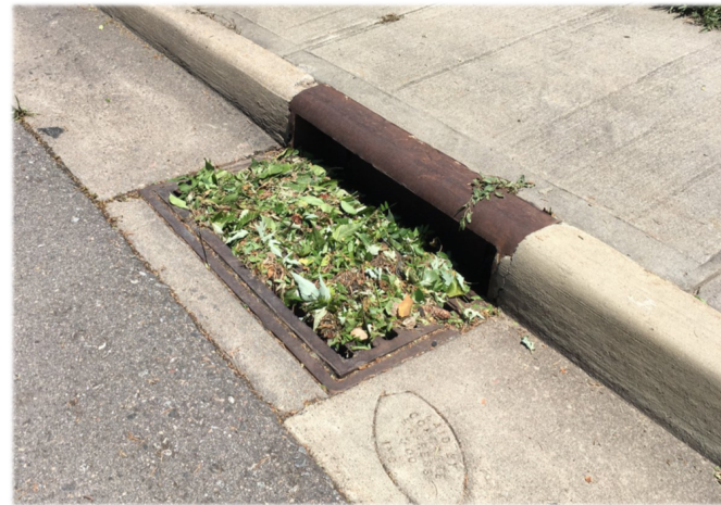
Figure: Clogged Inlet
