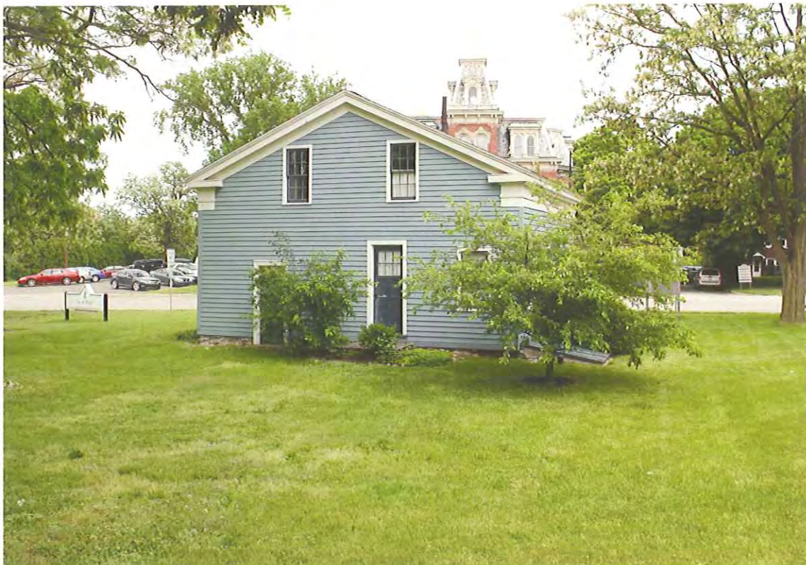
Towner House 303 N. Huron Street - Back View - West side
