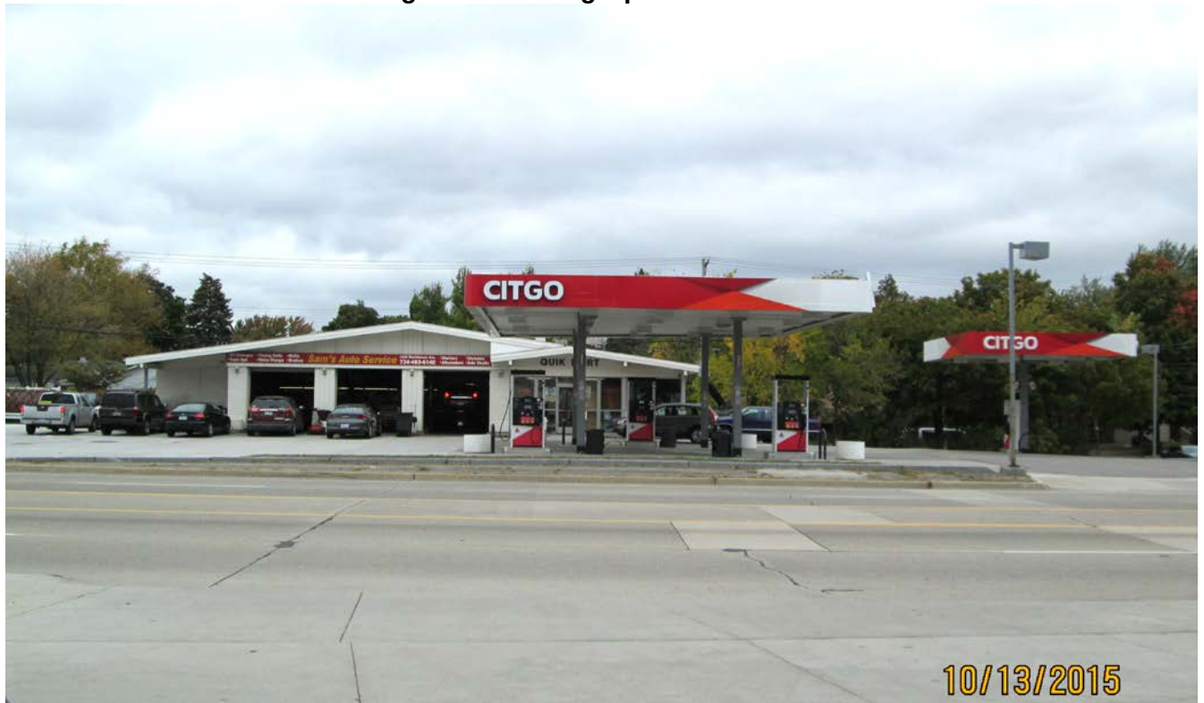
Figure 3: Photograph of Site
