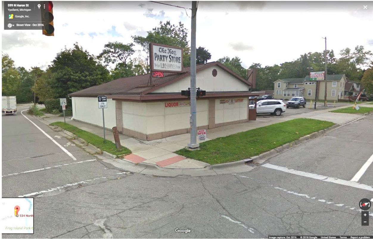
Figure 3: Google image of site-looking southeast
