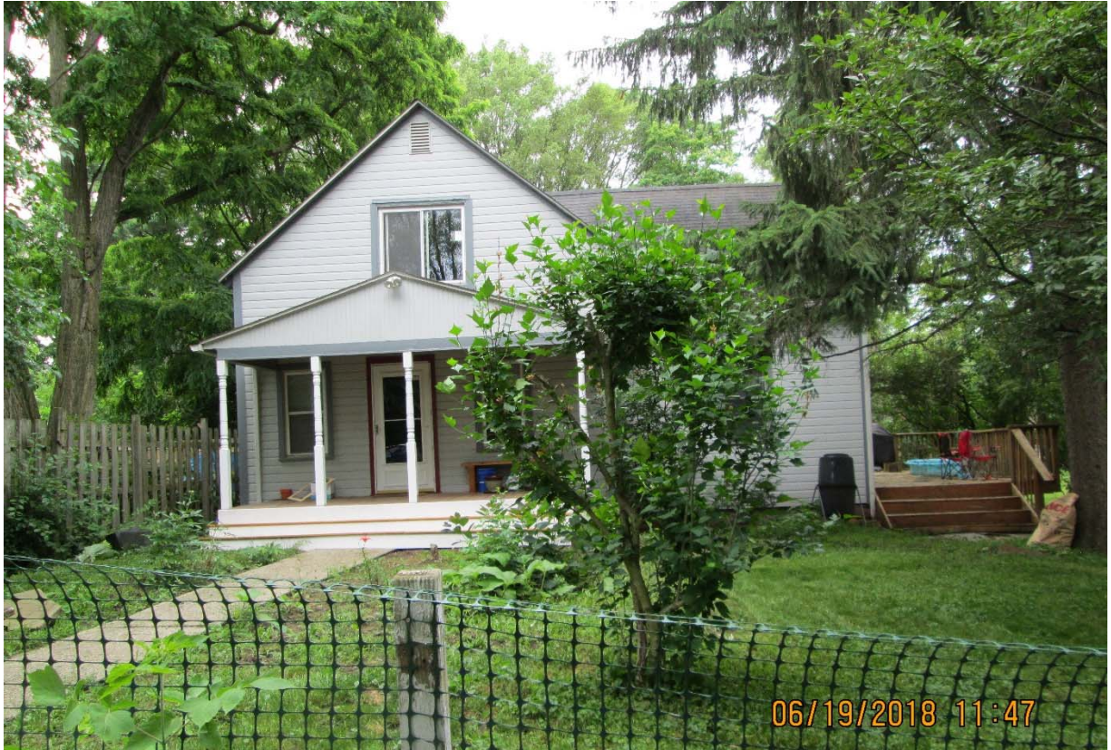
Figure 3: photograph of structure, south of Photo St.
