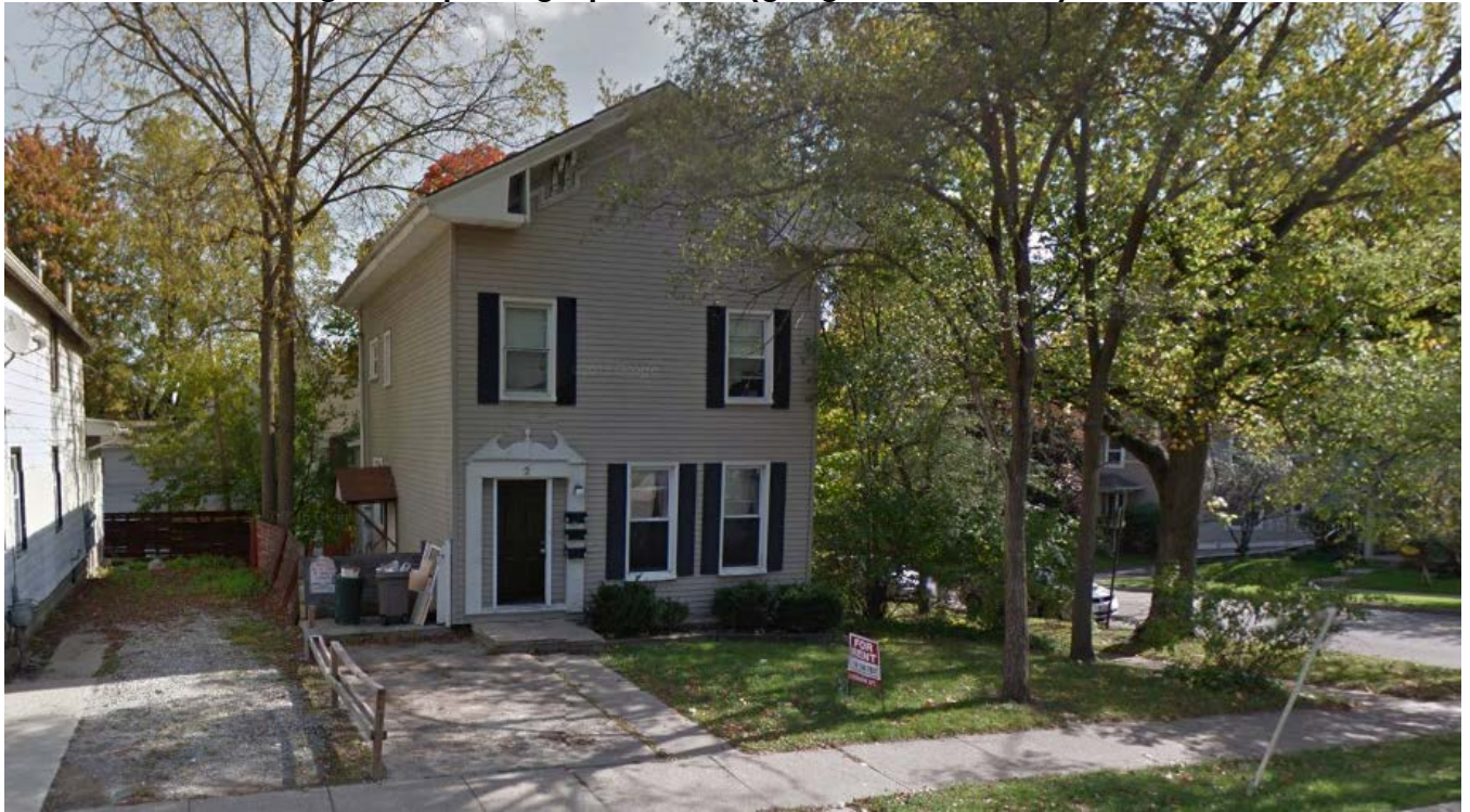
Figure 3: photograph of site (google street view)
