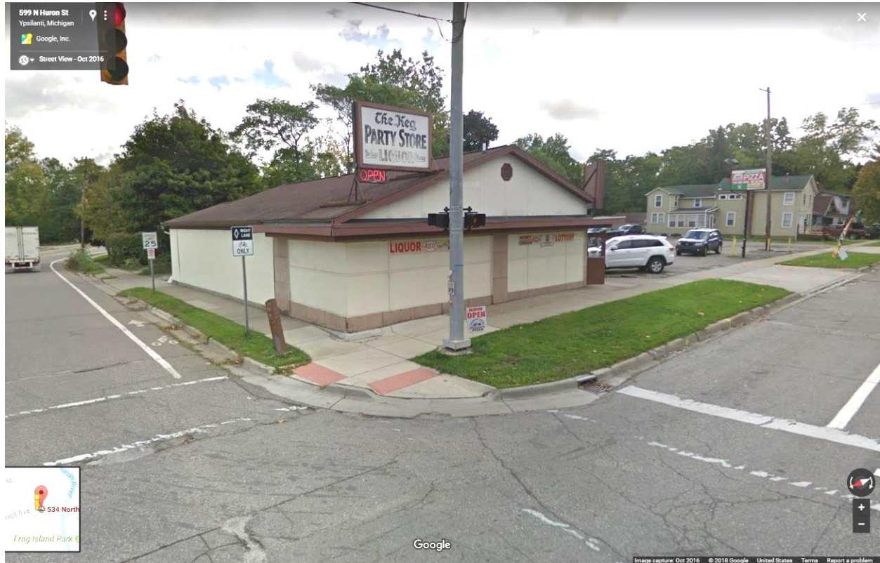
Figure 3: Google image of site-looking southeast
