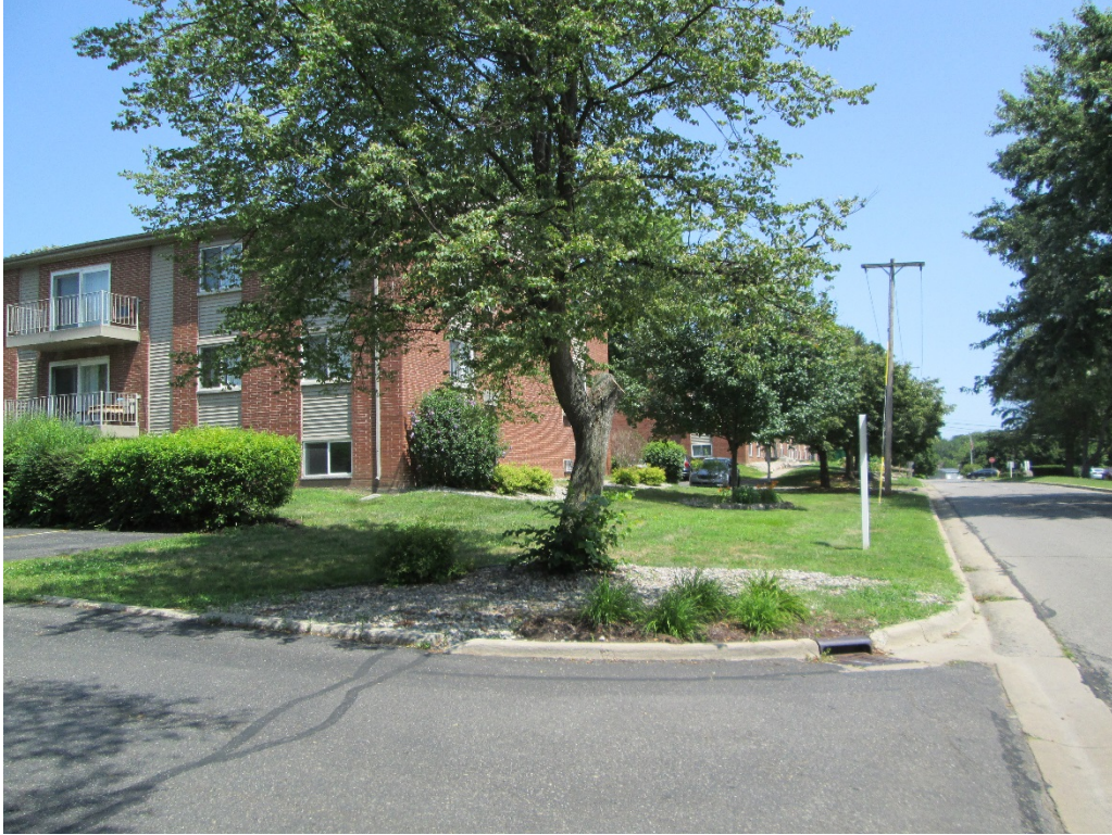
Figure 3: 772 Green Rd, facing east-northeast from the main entrance
