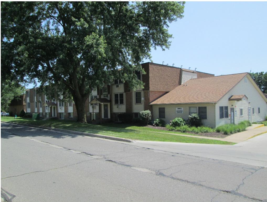
Figure 10: 799 Green Rd, facing southeast to east half of property, from Green Rd entrance
