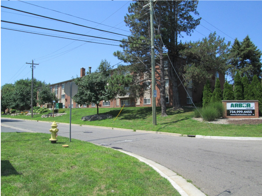
Figure 4: 772 Green Rd, facing northwest from Green and LeForge Rds, showing Green Rd frontage
