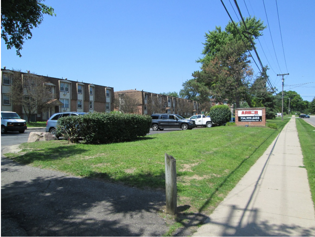
Figure 13: 799 Green Rd, facing northwest to LeForge Rd frontage
