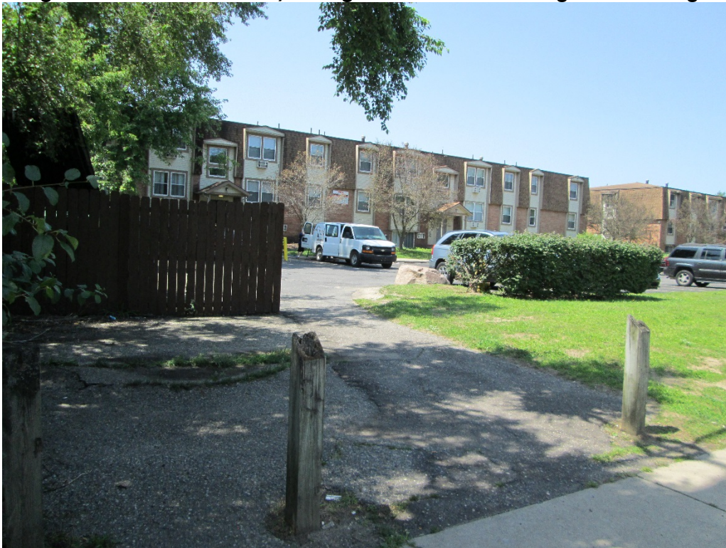
Figure 12: 799 Green Rd, facing west-northwest to LeForge Rd entrance
