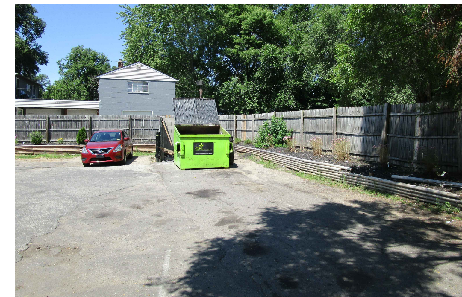
7 Existing Image - Dumpster Location E100
