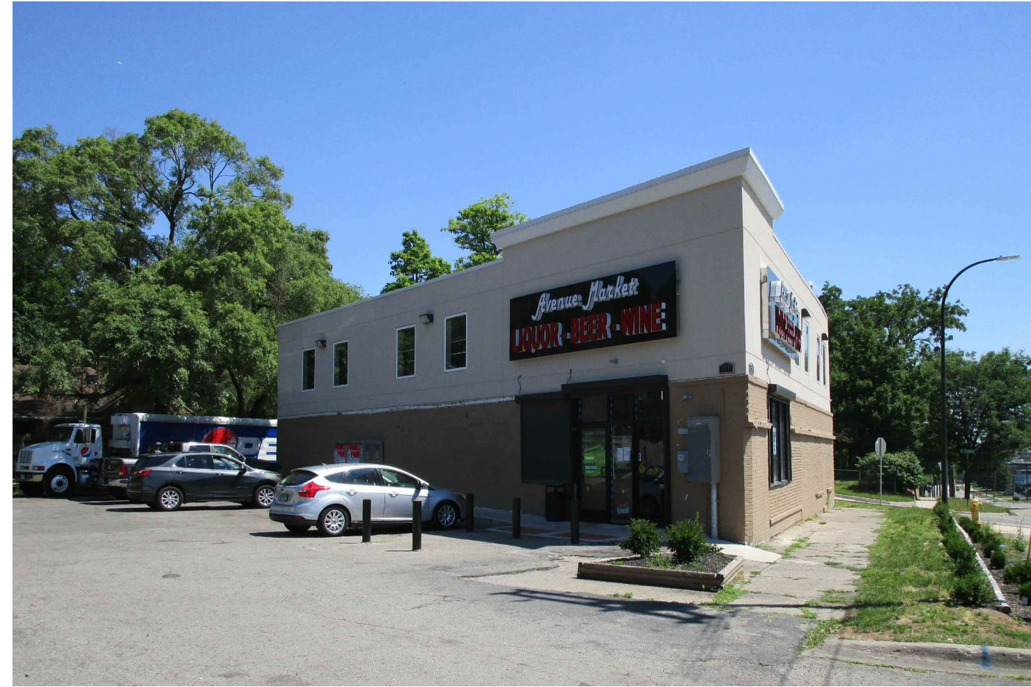
2 Existing Image - Entry Facade E100
