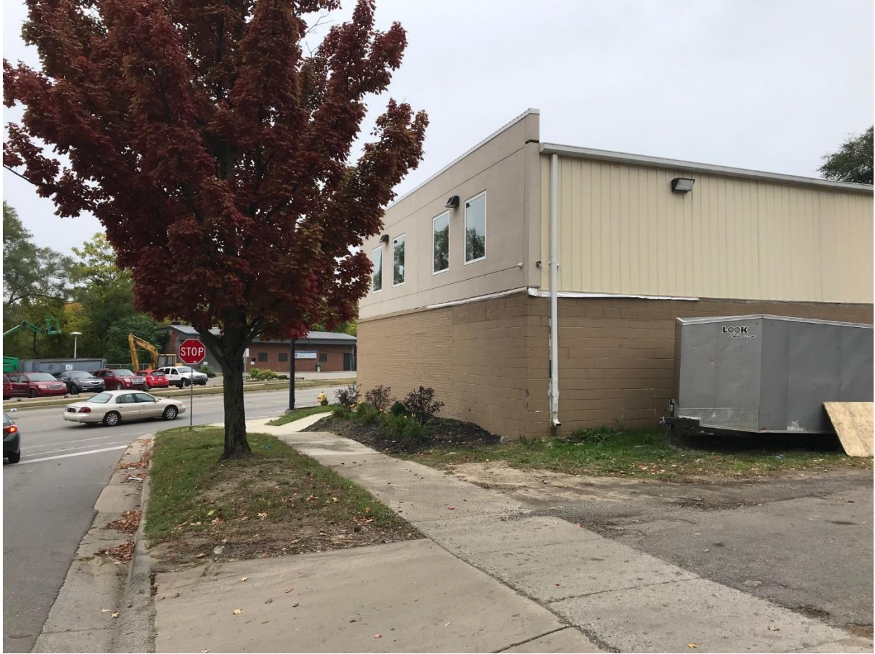
Figure 6: Photo of East Facade (October 14, 2020)
