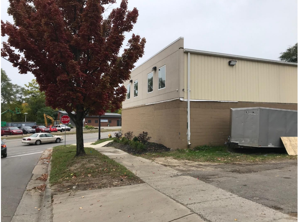
Figure 6: Photo of East Facade (October 14, 2020)
