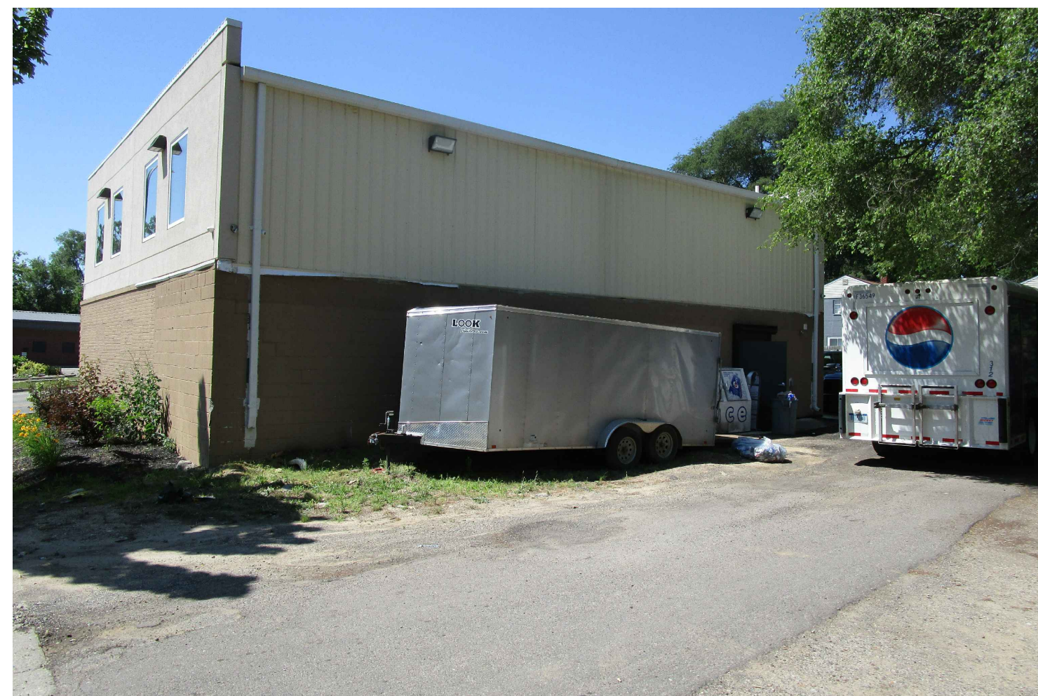
5 Existing Image - Rear Facade E100
