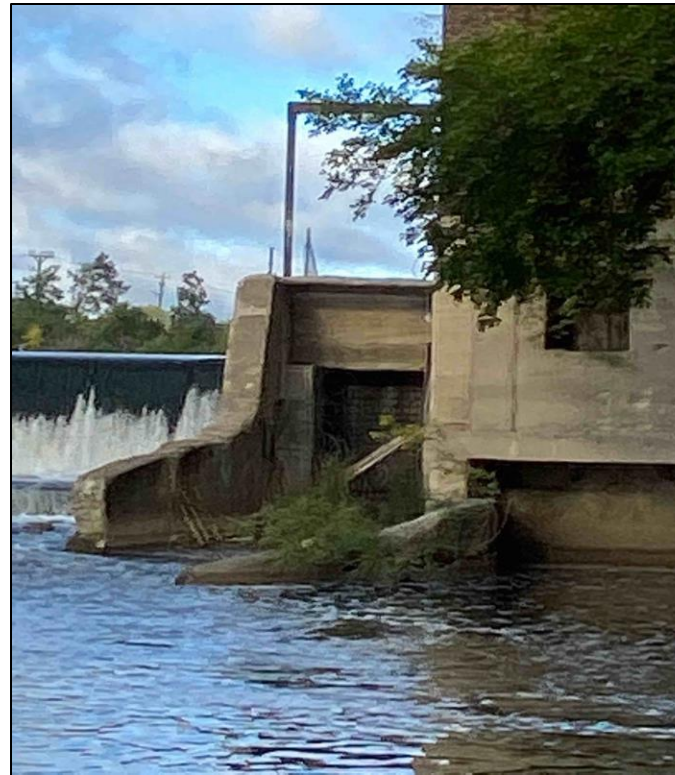
Stoplog Auxiliary Spillway
