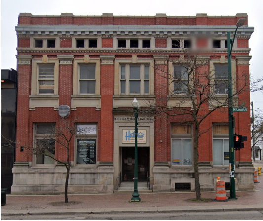
133 West Michigan Ave. was deemed noncontributing in 1989 due to extensive alterations. This building, like many others, has since been restored (Google Street View, 2023).
