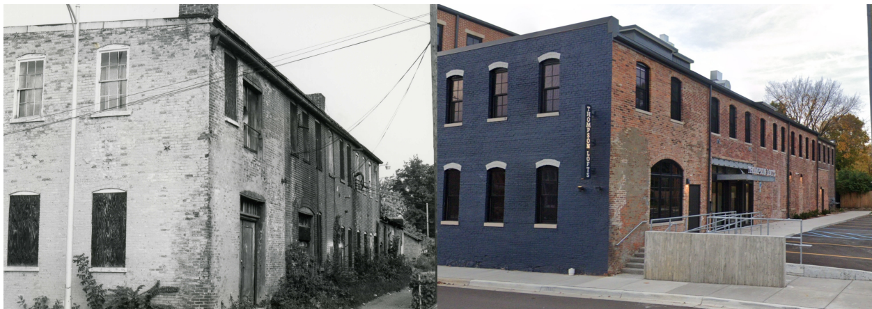
Left: southeast corner of Thompson Block, 400–410 N. River St. from the Ypsilanti Historic District National Register nomination; right, the same corner in 2020 (Google Street View). Built in 1861, it caught fire in 2009. Rehabilitation was completed in 2021.
