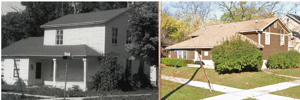
Left: 419 N. Hamilton from the Ypsilanti Historic District National Register nomination; right: the same house in 2020, showing extensive alterations made in 1977 (Google Street View)
