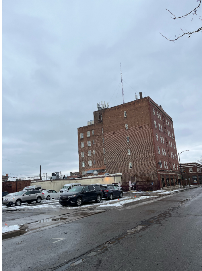
Figure 4: Photo of Site from N Washington St
