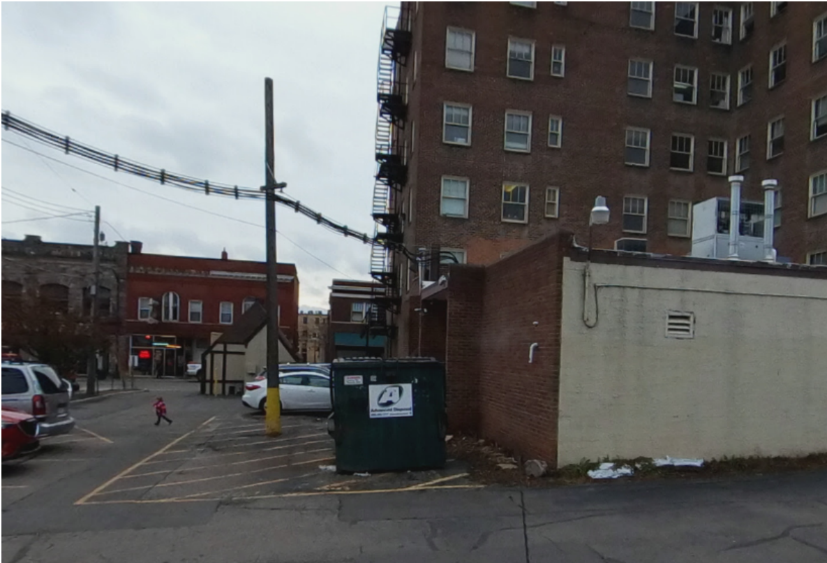
Figure 10: Existing Unscreened Trash Receptacle
