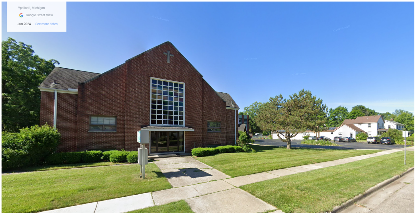
Figure 3: Photo of Site from E. Forest Ave
