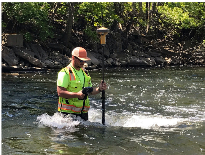
Inter-Fluve's Garrett Shear collecting survey data downstream of Pen Dam in the Huron River in 2021.
