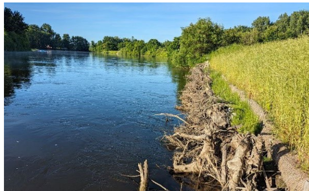
Toewood and bioengineered lifts, designed and constructed by GEI staff on the Muskegon River.
