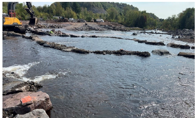
Repubilic Dam rock rapids construction. The "sine-wave" configuration for boulder placement is the first of its kind constructed in Michigan and increases aquatic organism passage and rapids stability on larger rivers.
