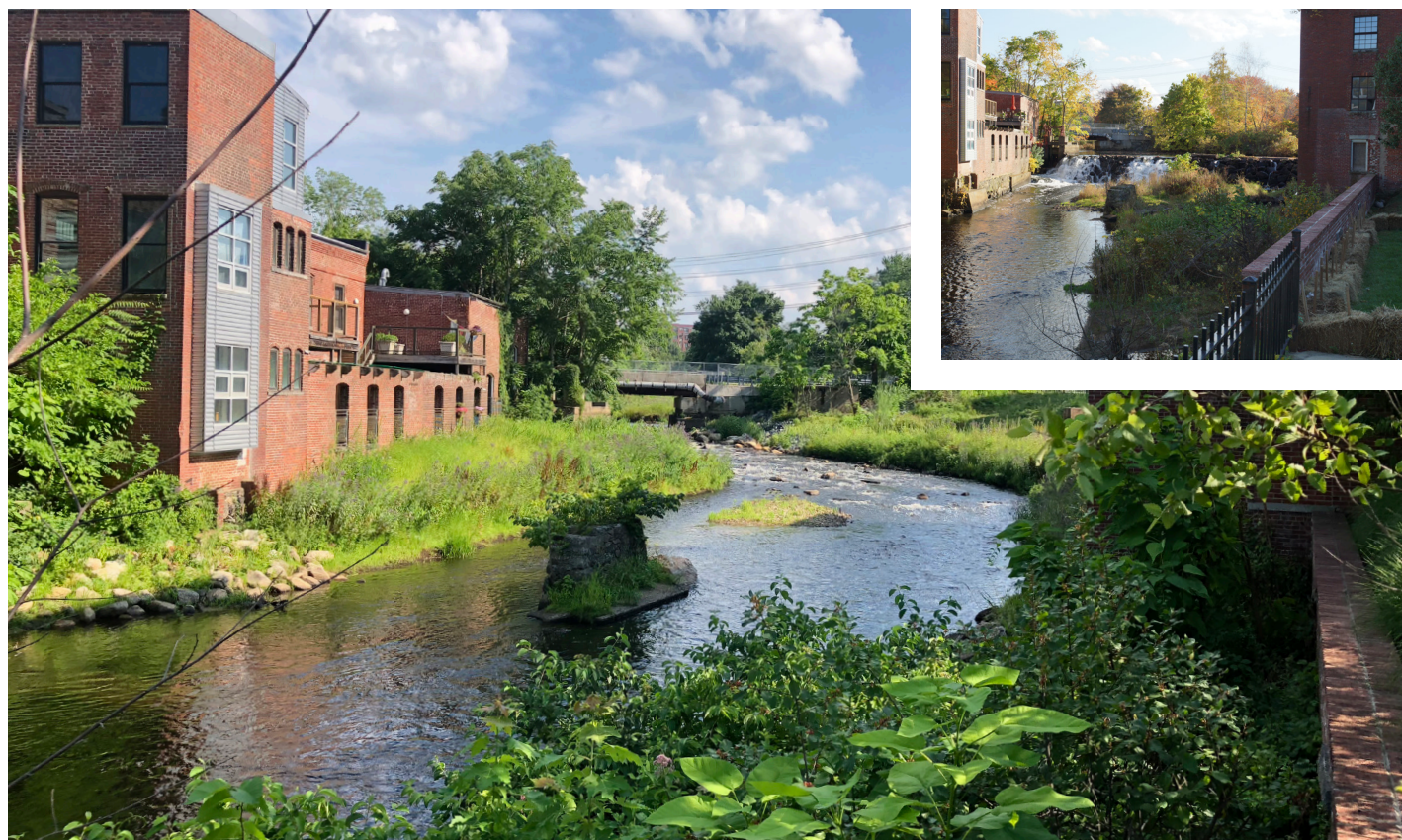
Shawsheen River, MA. Inter-Fluve led the removal of the Marland Place Dam, shown before (inset) and after removal.
