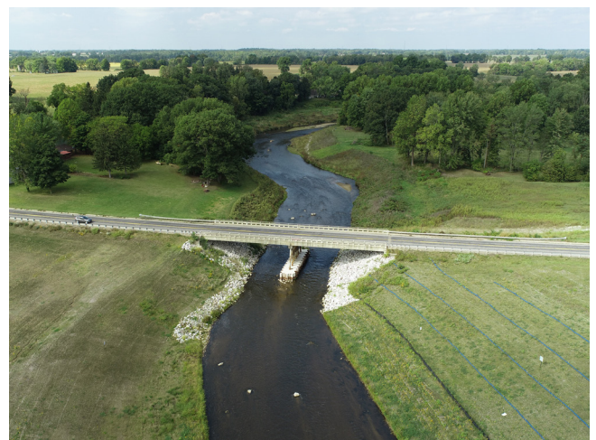
Dowagiac River, MI. Drone images of the Pucker Dam site before, during, and after removal. Photo credit: Jeff Dunlap, City of Niles.
