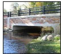
Figure 4-D: Three-sided box bridge
