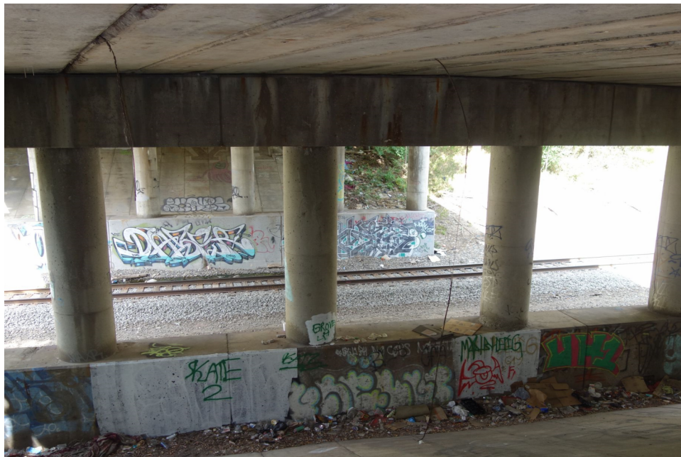
Typical face of pier
