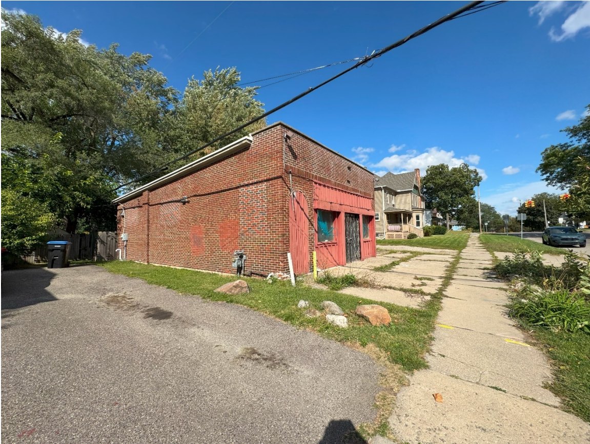
Figure 3: 908 N. Congress Site Conditions - Facing Northeast (September 2025)
