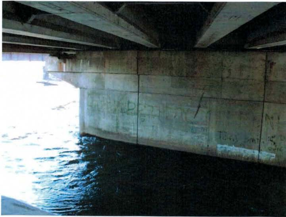
Pier, West Face, North Half
