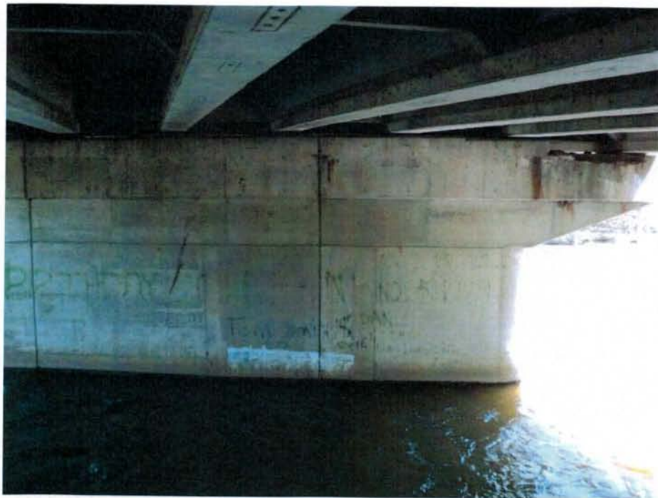
Pier, West Face, South Half
