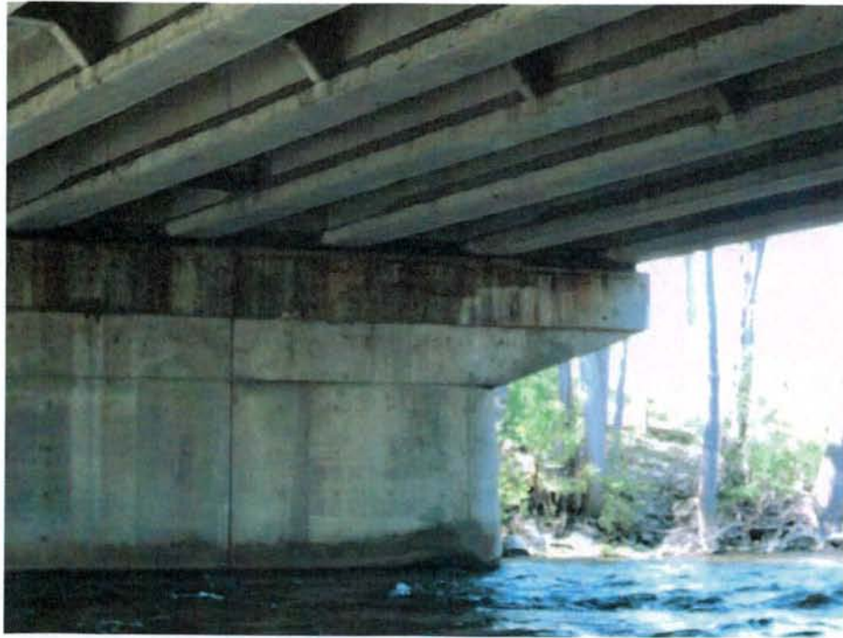
Pier, East Face, North Half
