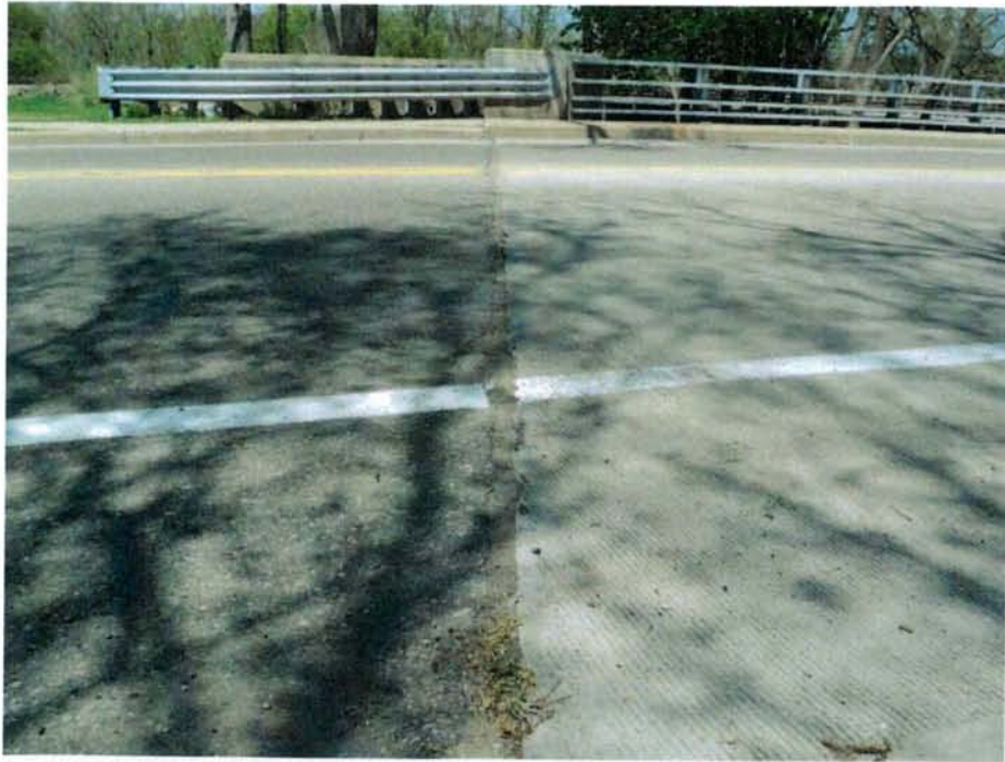
West Reference Line Joint
