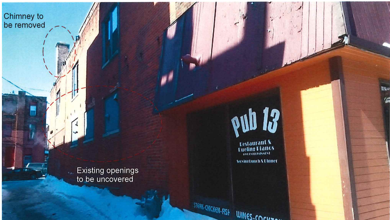
Existing Alley View: note chimney and boarded-up windows
