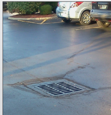
Runoff from coal-tar-sealcoated pavement goes down storm drains to receiving water bodies. The runoff contains high concentrations of PAHs and related chemicals that can harm aquatic life. 16
