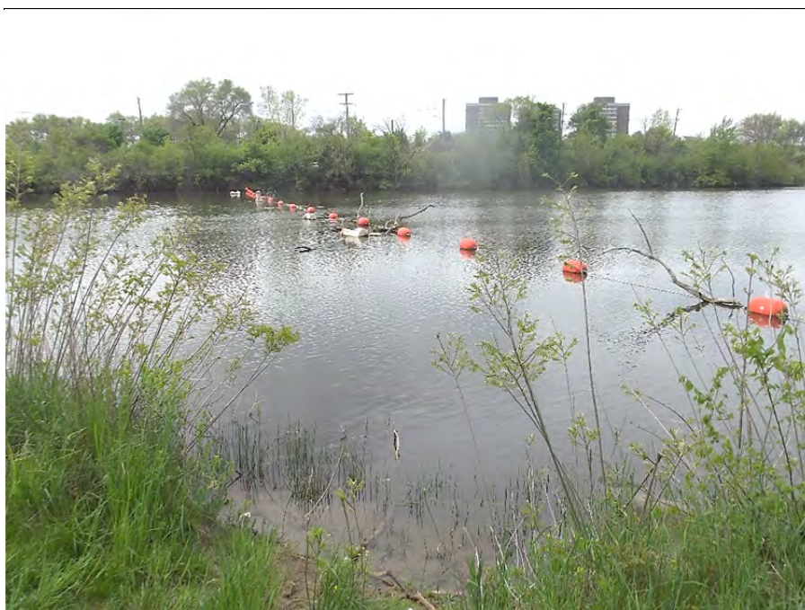
Photograph 28 – Impoundment viewed from the left embankment Note the cable buoy barrier
