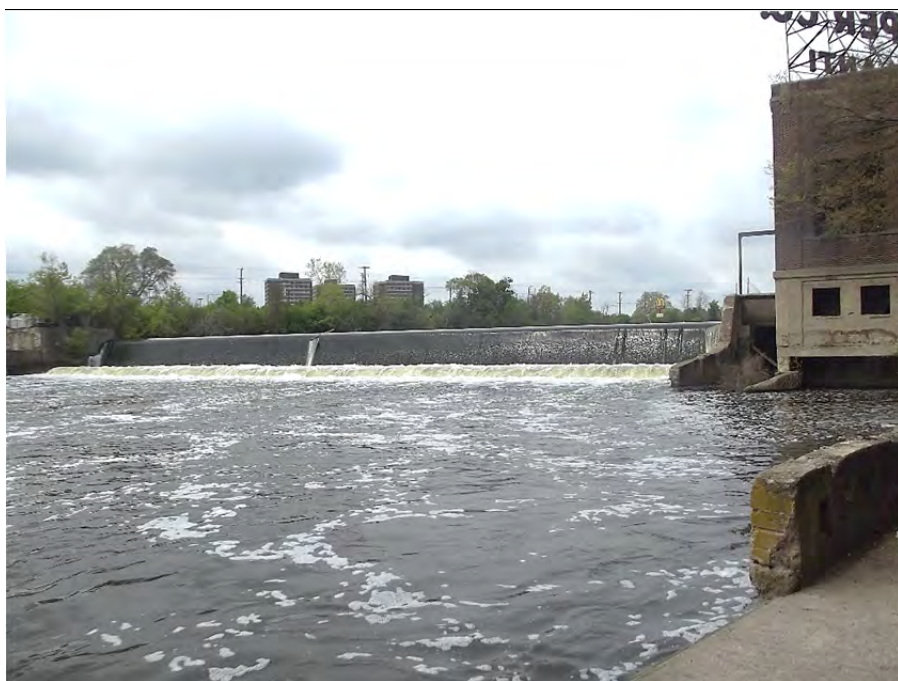
Photograph 12 – Principal spillway viewed from downstream
