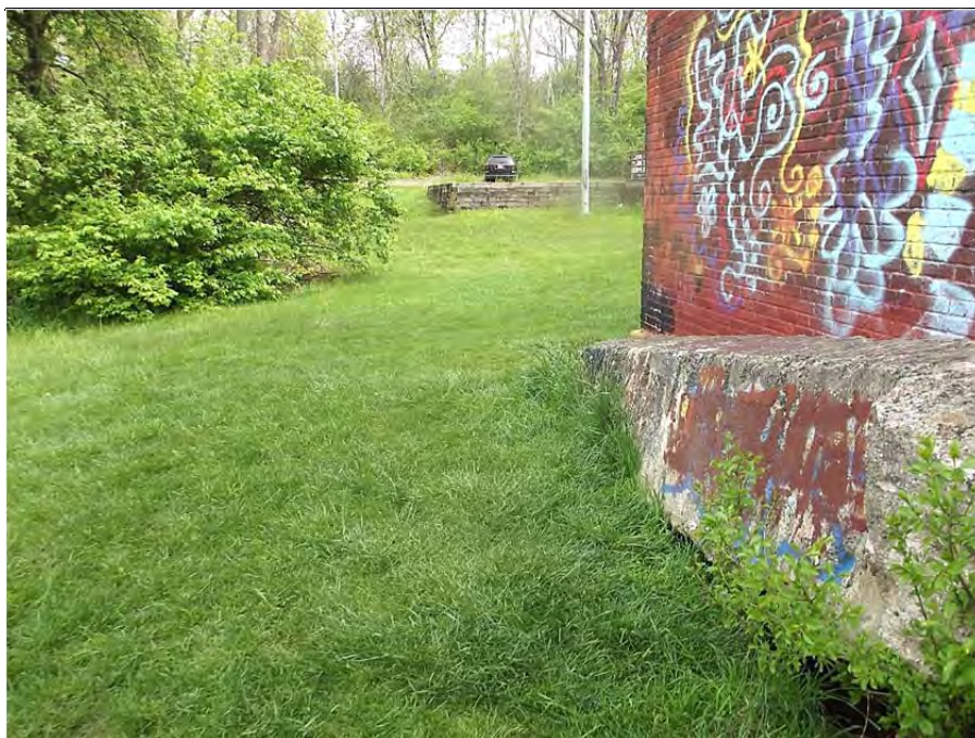
Photograph 5 – Crest of the left embankment viewed from the right
