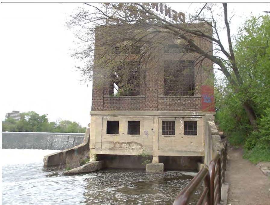
Photograph 23 – Powerhouse viewed from downstream
