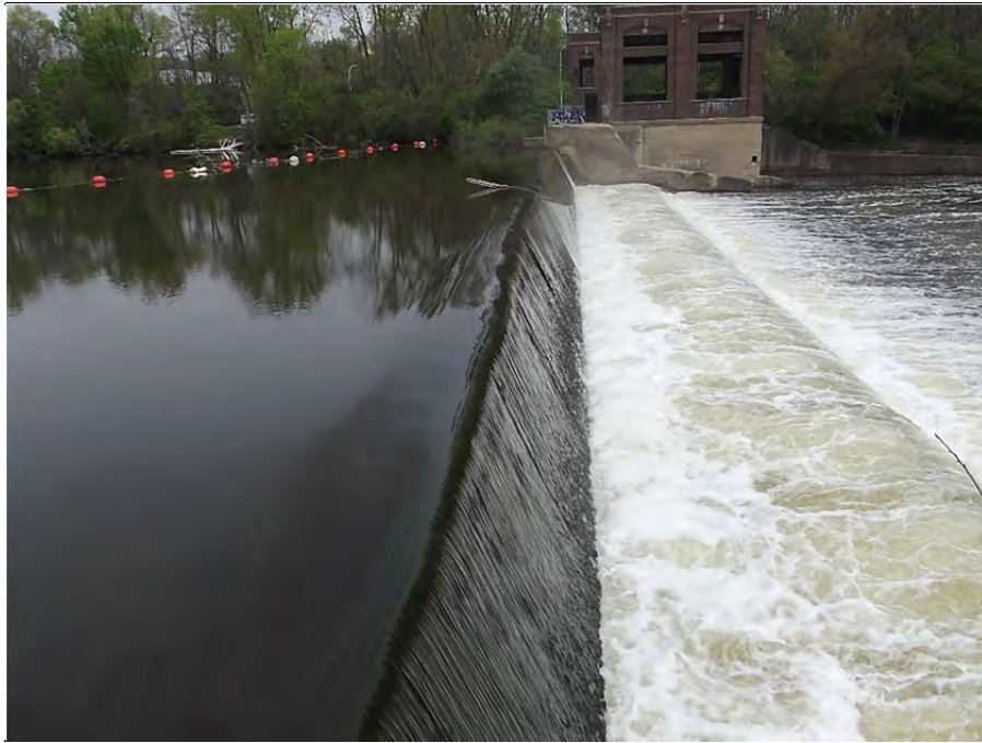
Photograph 13 – Principal spillway crest viewed from the right
