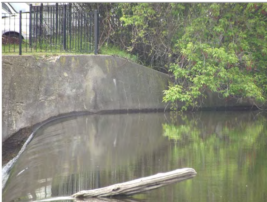
Photograph 17 – Upstream left principal spillway abutment wall
