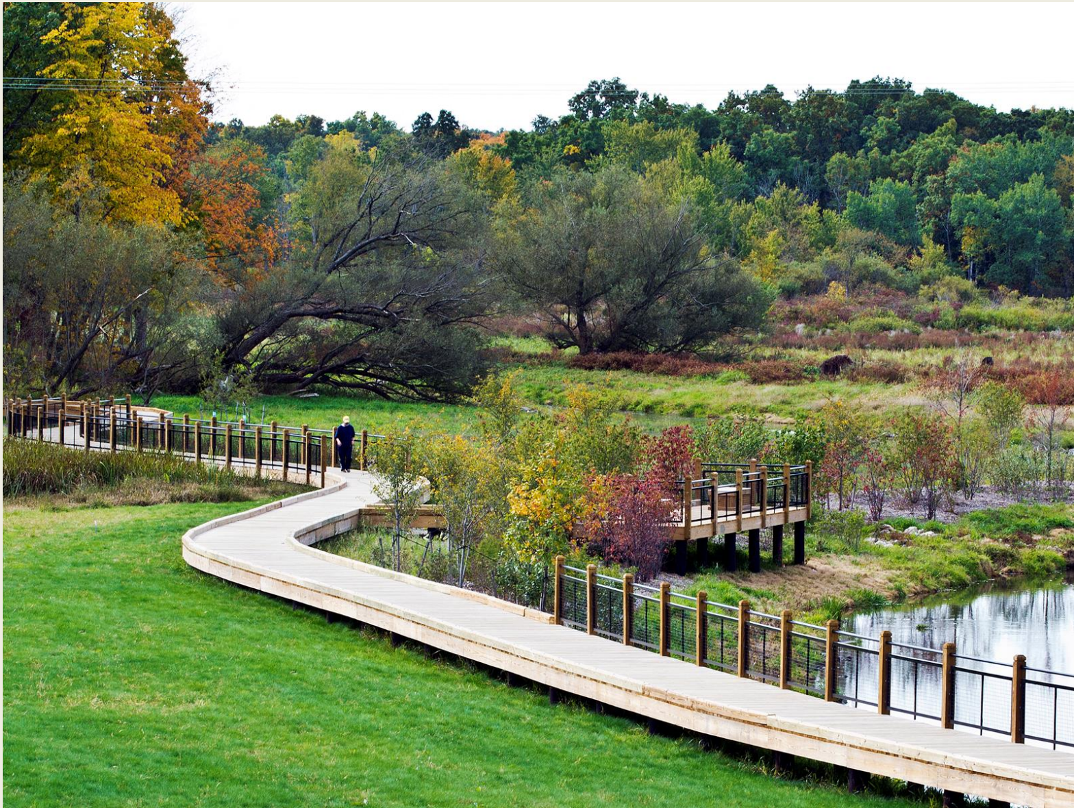
Mill Creek Dam removal and restoration in Dexter, Michigan
