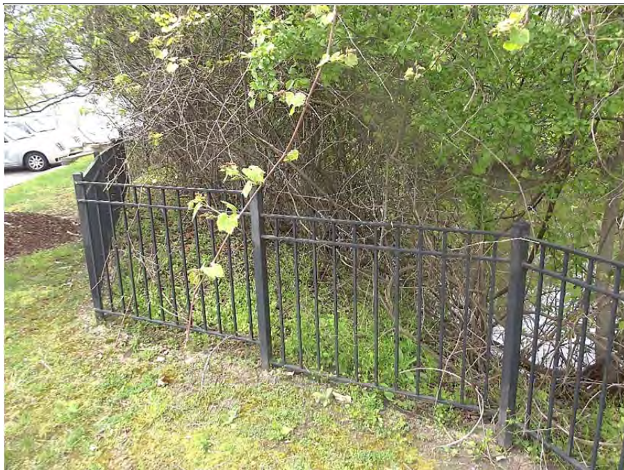
Photograph 8 – Upstream face of the right embankment viewed from the left Note the trees and brush
