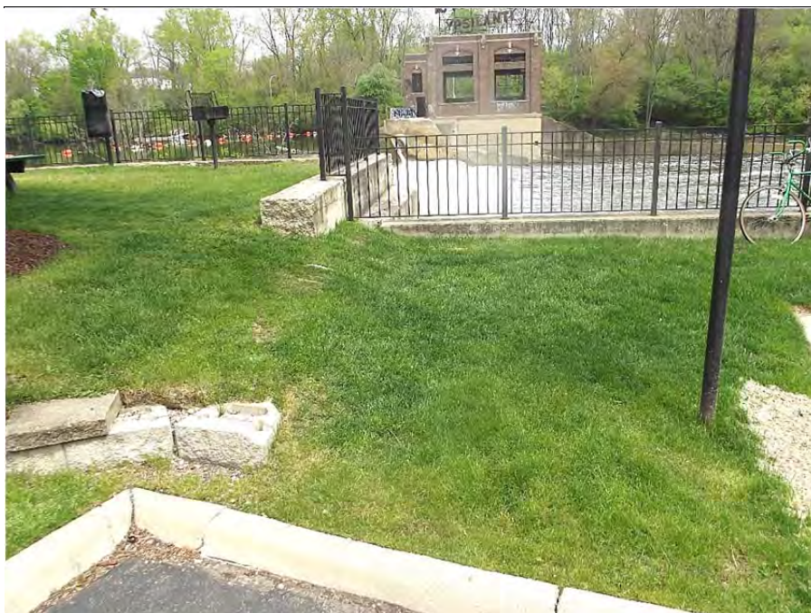
Photograph 10 – Downstream face of the right embankment viewed from the right
