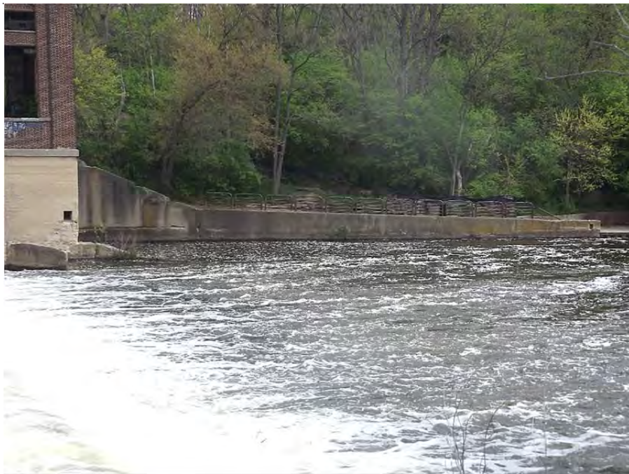
Photograph 26 – Downstream left abutment wall of the powerhouse
