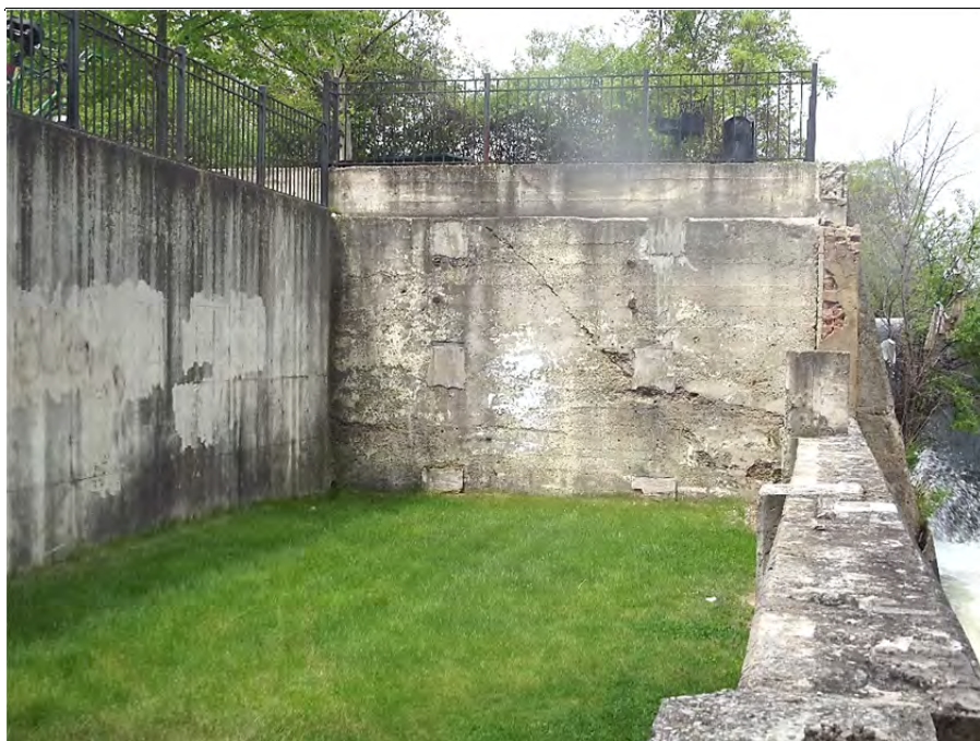
Photograph 11 – Downstream face of the former mill foundation at the right embankment
